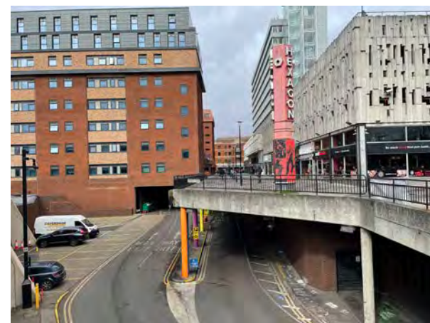
East of the Hexagon is the pedestrianised raised podium, and Broad Street Mall.
