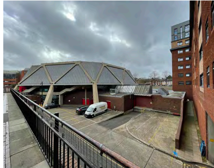
Approach to the Hexagon from podium level, Queens Walk
