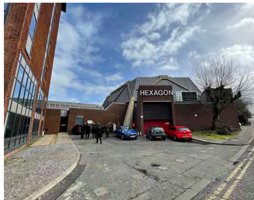
Rear of the Hexagon, from the IDR slip-road
