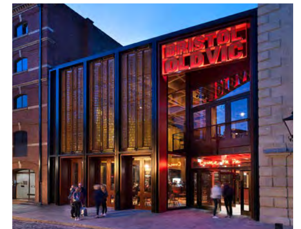
Haworth Tompkins transformed the foyer arrival sequence, remodelling the foyer as an extension of the public realm
