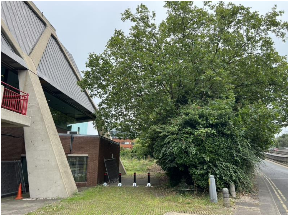
Figure 4: Looking southeast towards the existing access road that will be utilised during development. Pruning of T2, T3 and S6 is required to provide adequate clearance, as can be seen in this image.
