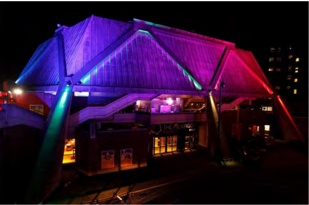
Existing Hexagon theatre’s lighting
