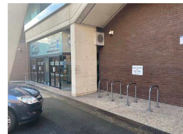
Fig.4 Existing cycle stands under cover
