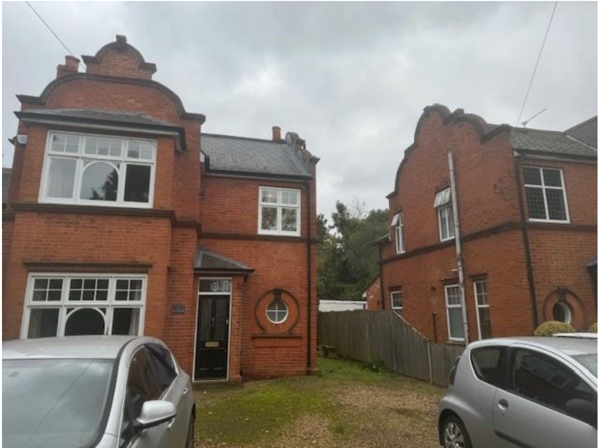
Site Visit Photos taken on the 16 th of October 2024
