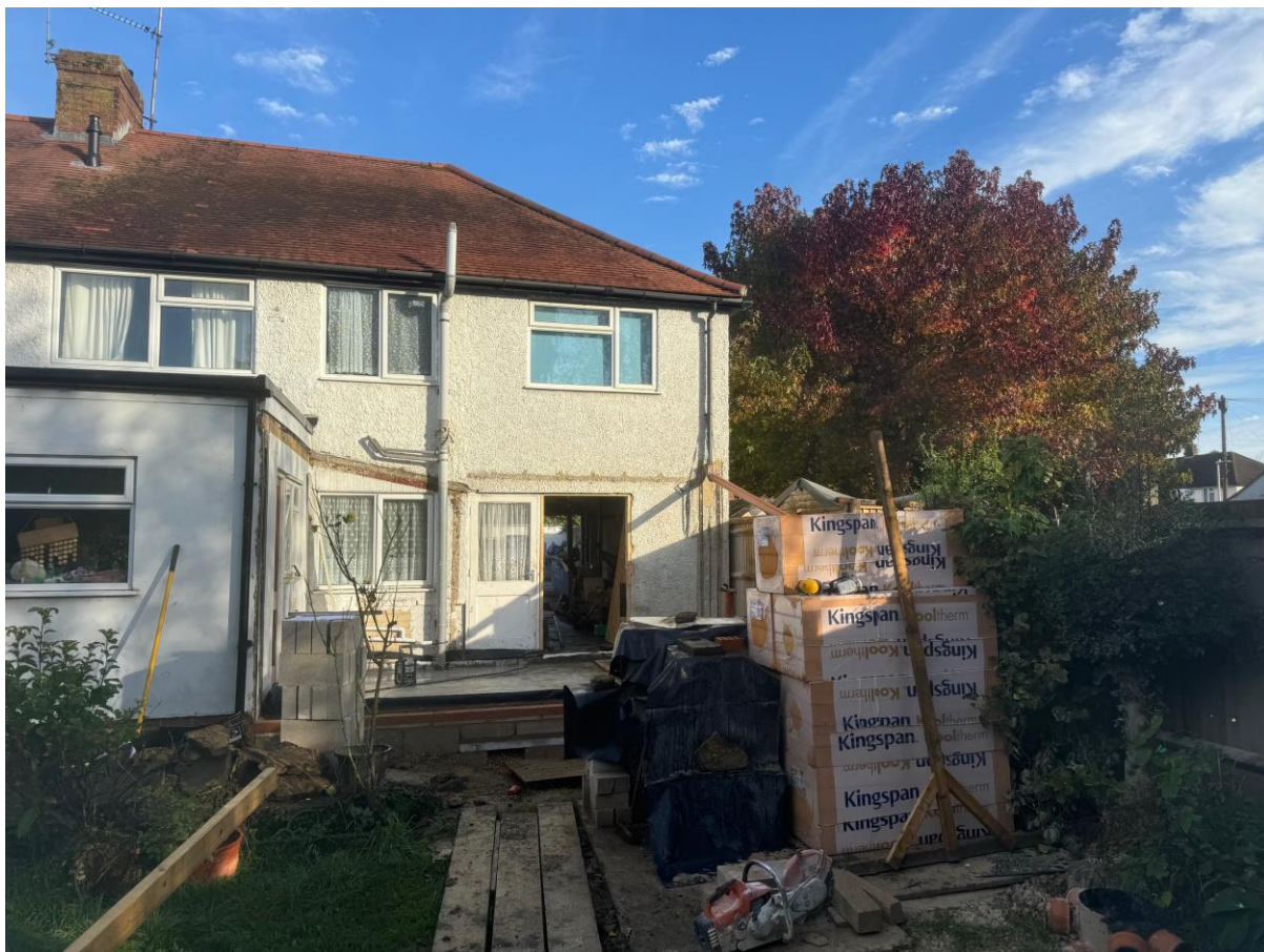
Site Visit Photos as taken on 17 th of October 2024
