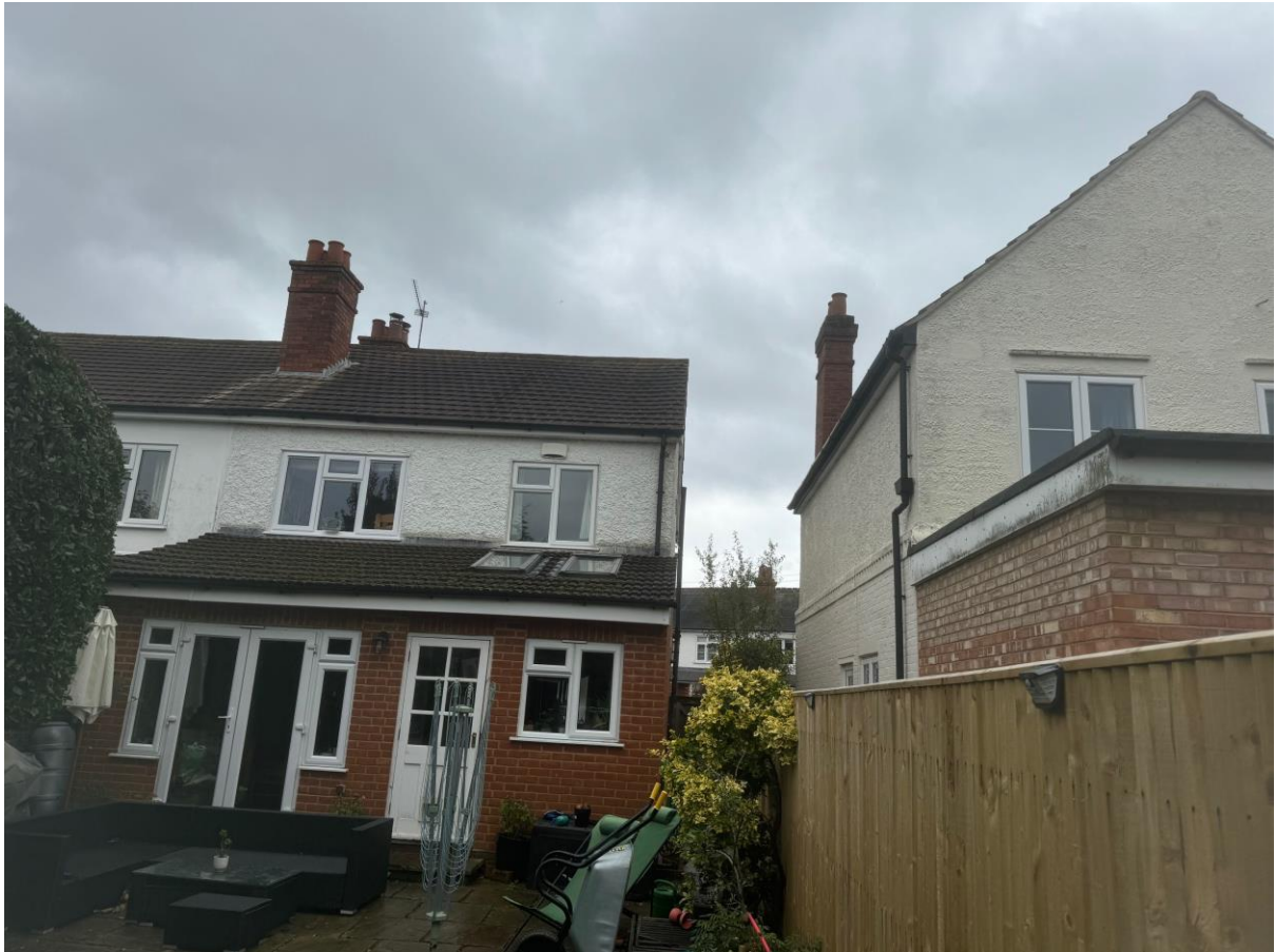
Site Visit Photos taken on 16 th of October 2024
