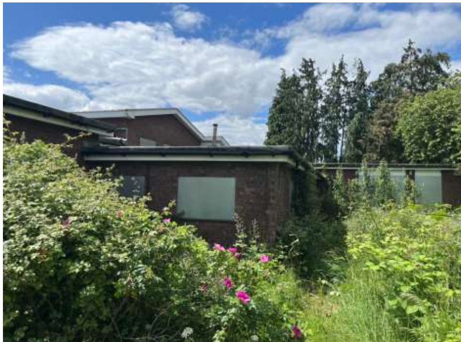
Figure 2: Existing building looking from the north east
