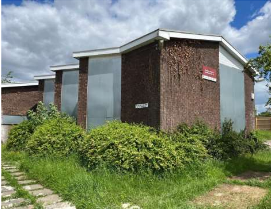
Figure 1: Existing building looking from the south east
