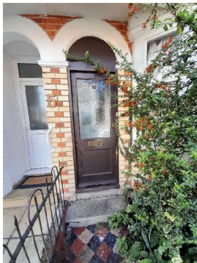
Existing outer front door
