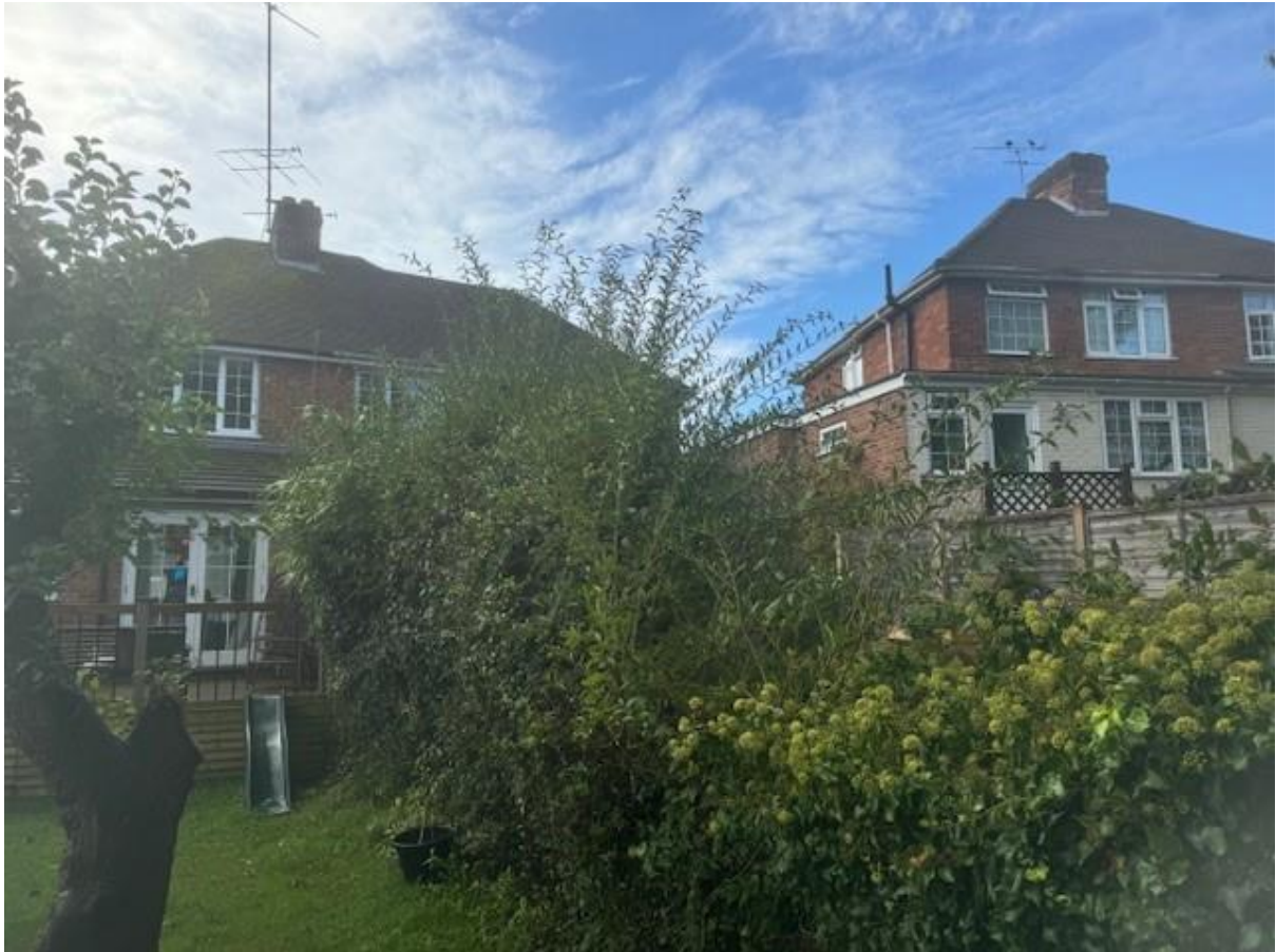
Site Visit Photos taken on 7 th of October 2024
