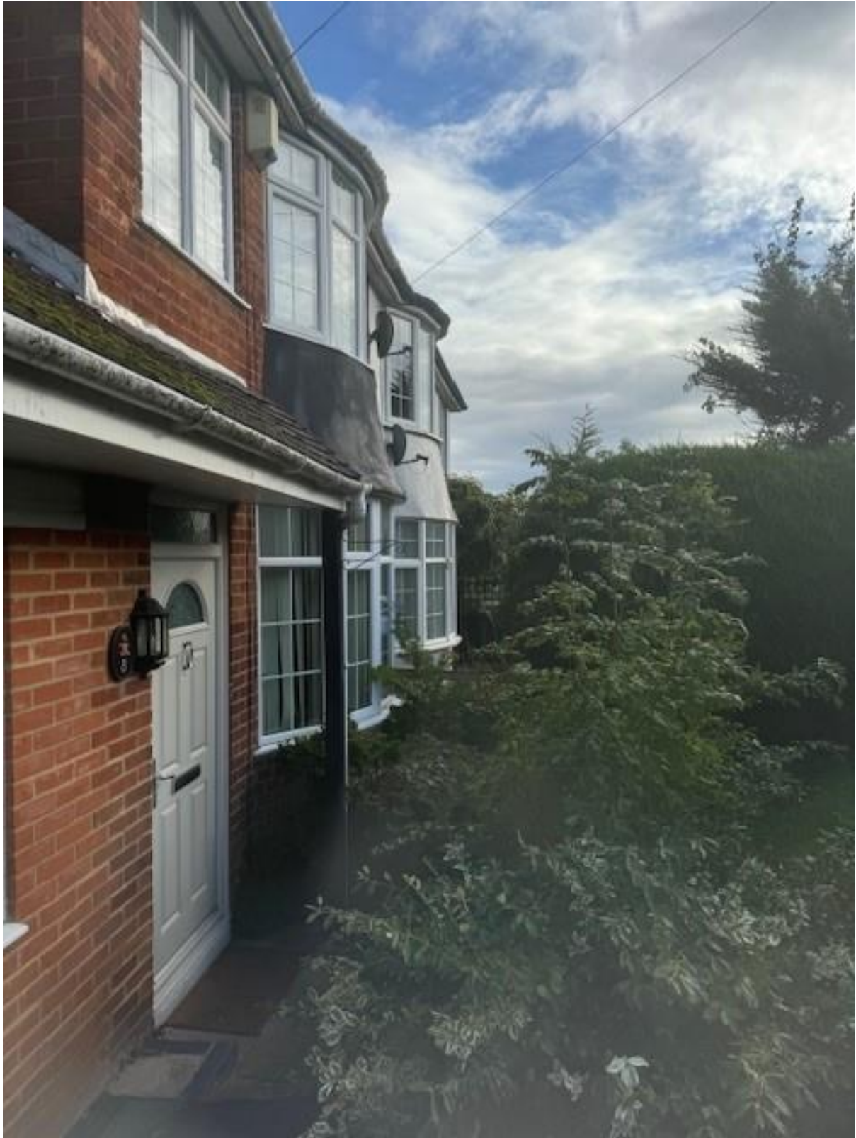
Site Visit Photos taken on 7 th of October 2024
