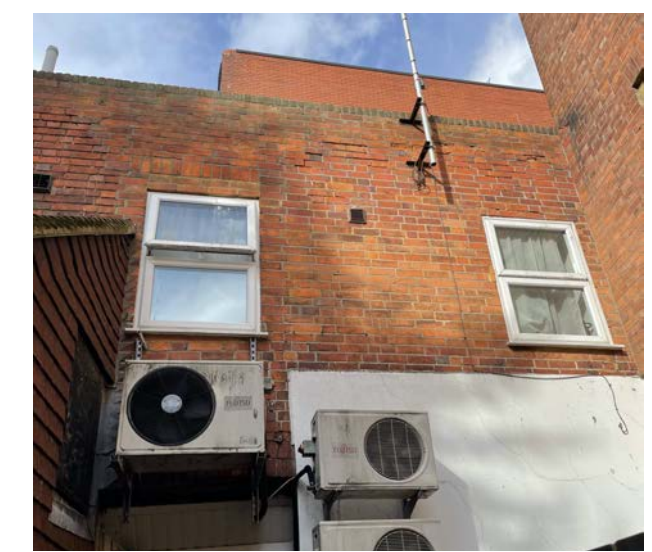
Photo of Existing rooms 03 and 04 windows
