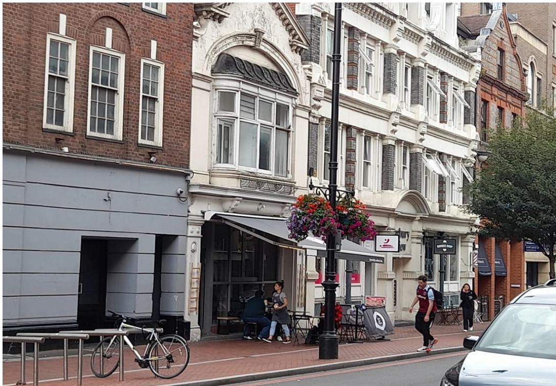
Fig. 1: View, looking north-west, of the western side of Blagrove Street, with No. 7 (centre) and surrounding buildings.
