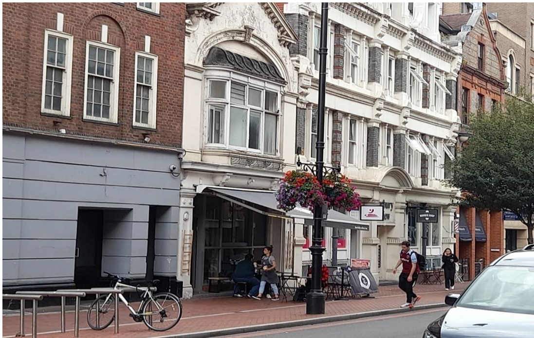
Fig. 18: View, looking north-west from the Grade II-listed Concert Hall, towards No. 7 Blagrove Street.
