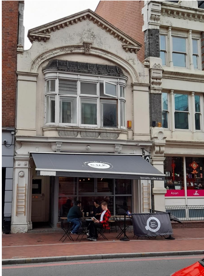
Fig. 5: View, looking west, of the street frontage of No. 7, Blagrove Street.
