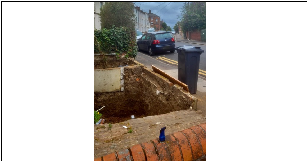
Figure 4 Excavations for front light well (from Jesse Terrace)
