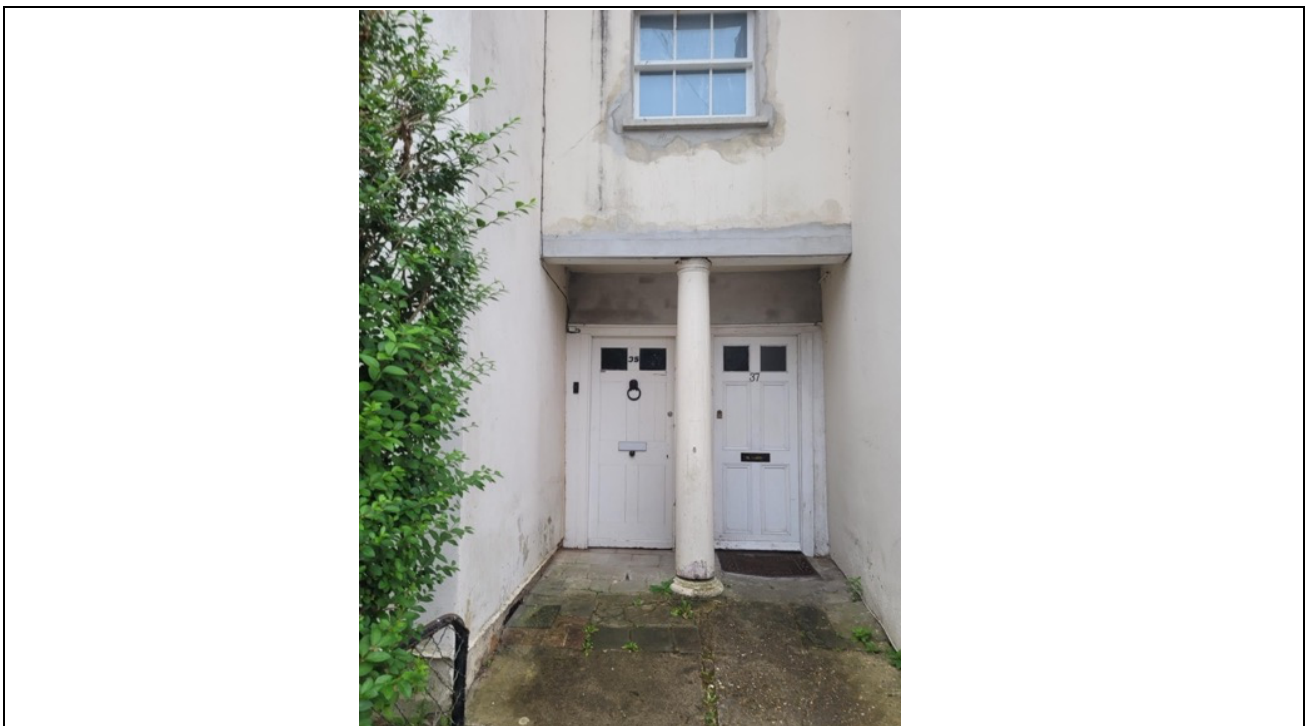
Figure 3 Entrance doors to 35 & 37 Baker Street - note area above front doors
