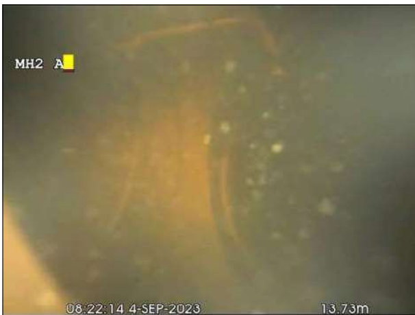
Photo: 36_9a, 00:00:00 13.7m, Manhole Remark: Chamber visible
