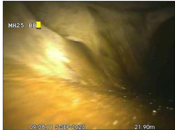
Photo: 363_7a, 00:00:00 21.9m, Manhole Remark: MH
