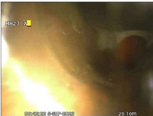
Photo: 314_11a, 00:00:00 26.2m, Manhole Remark: MH
