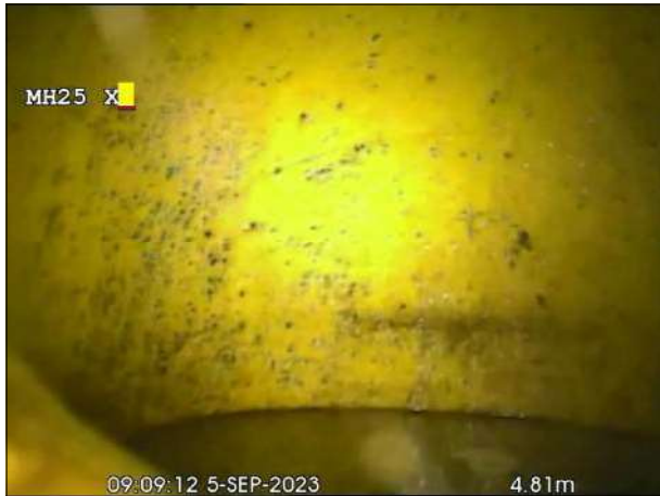
Photo: 349_3a, 00:00:00 4.8m, Manhole Remark:MH
