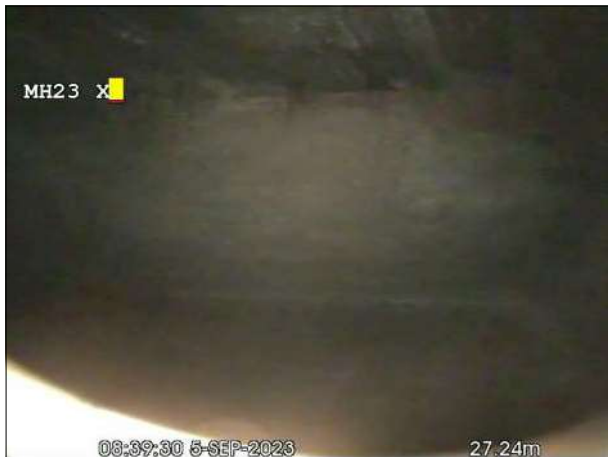
Photo: 35_6a, 00:00:00 27.7m, Finish Survey, Remark: Culvert
