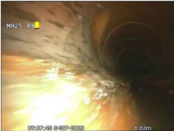
Photo: 360_3a, 00:00:00 6.7m, Junction at 10 o'clock, dia 150 mm
