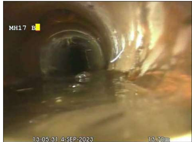
Photo: 244_7a, 00:00:00 14m, Junction at 12 o'clock, dia 100 mm
