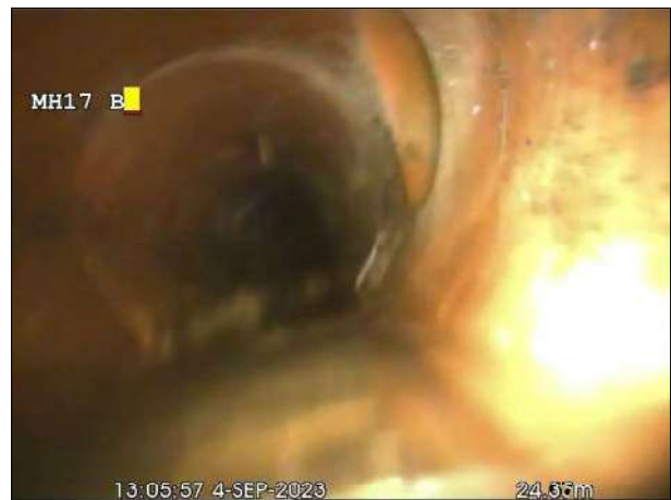
Photo: 248_11a, 00:00:00 24.5m, Junction at 03 o'clock, dia 150 mm
