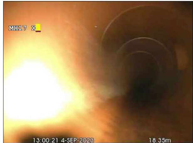
Photo: 232_4a, 00:00:00 18.5m, Junction at 03 o'clock, dia 100 mm
