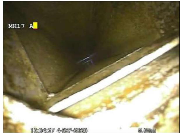
Photo: 231_7a, 00:00:00 5.85m, Finish Survey, Remark: DP
