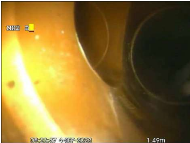
Photo: 3_4a, 00:00:00 1.5m, Junction at 11 o'clock, dia 80 mm
