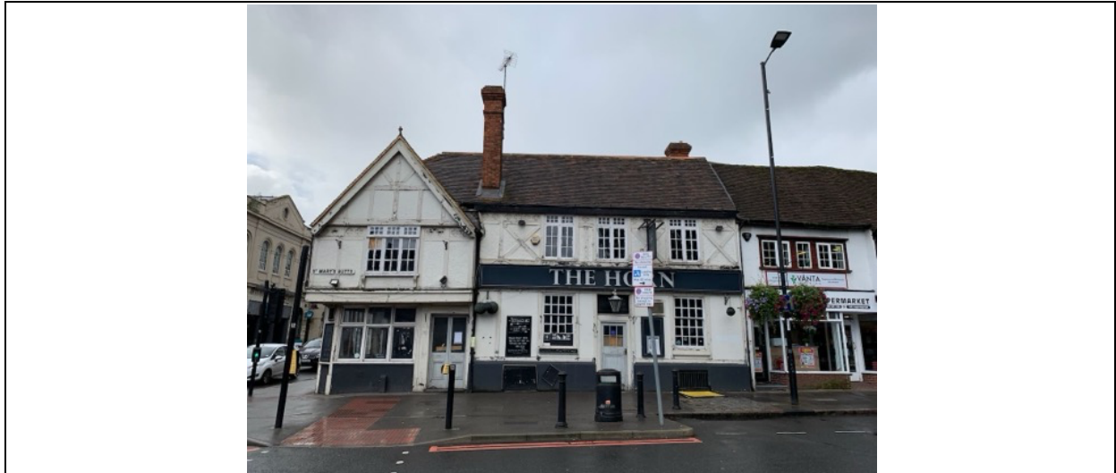
Figure 6 St Mary's Butts elevation October 2024. The original public house building to the right.
