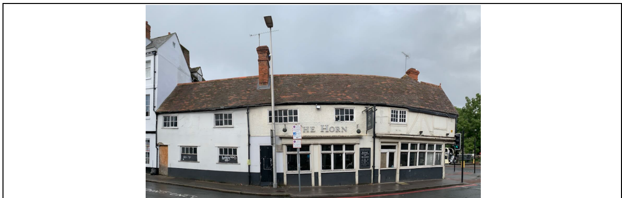
Figure 5 Panoramic photo of southern elevation of The Horn – from L to R - 6, 4, 2 Castle Street. October 2024.
