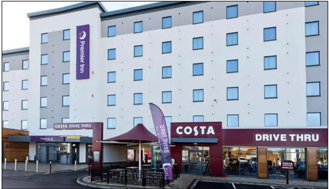
Figure 1 Reading South (Gateway, M4, J11) (Source. Premier Inn (2024))
