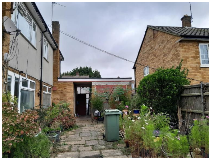
Fig1: Taken from the rear of the application site by the officer, 1 st October 2024.
