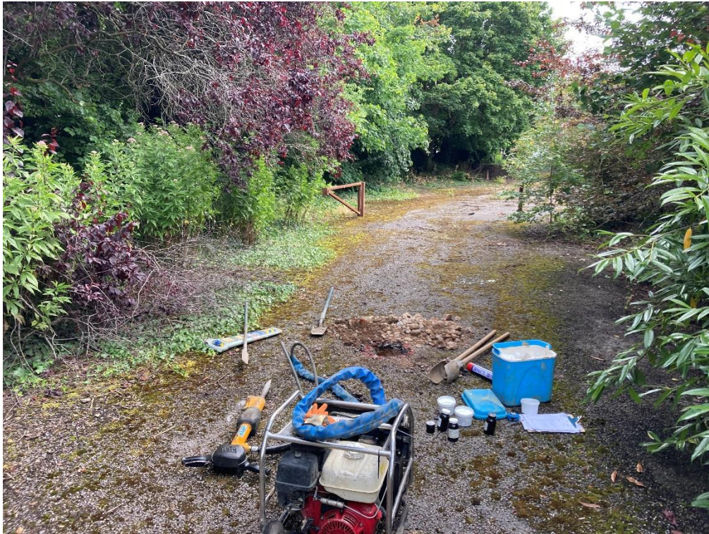
Hand-dug trial pit ('Sub-Base' Made Ground)
