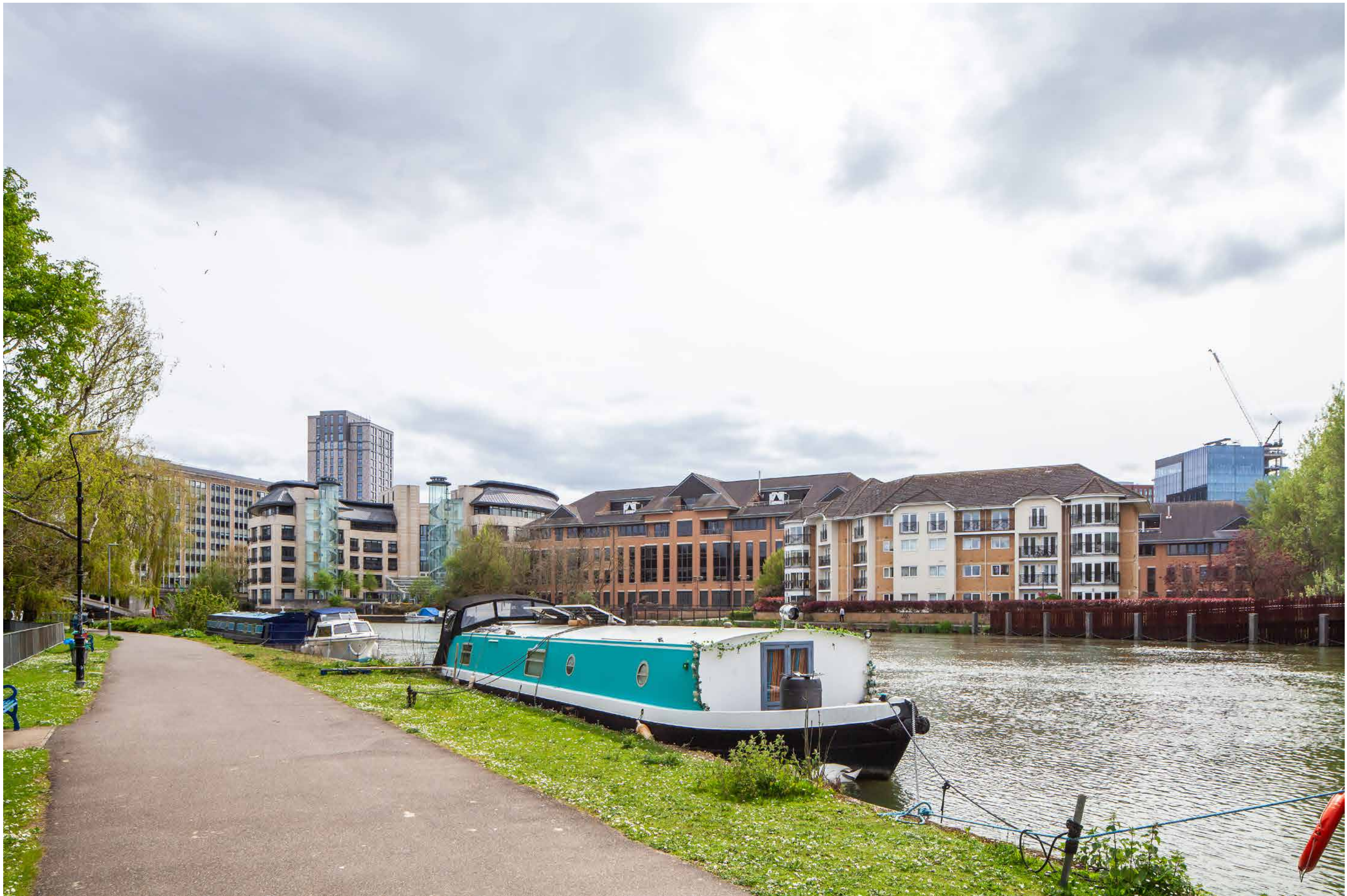
View 11: Existing (April '24)
