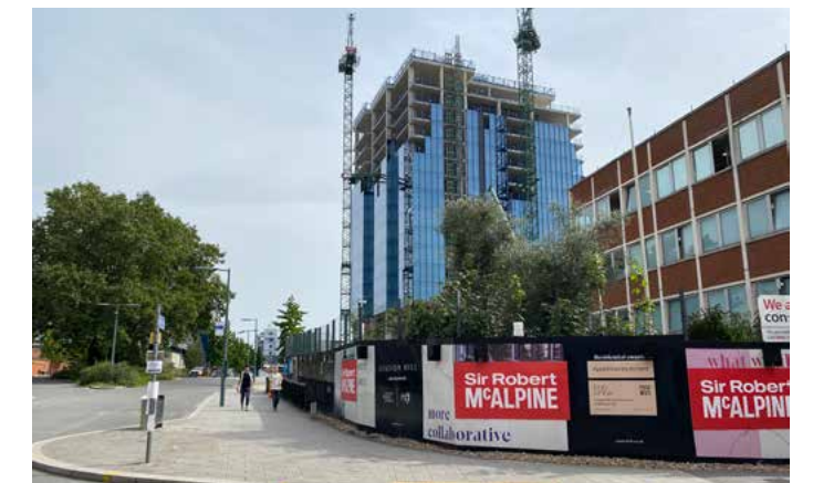
Photo 23: One Station Hill (under construction at time of capture)
