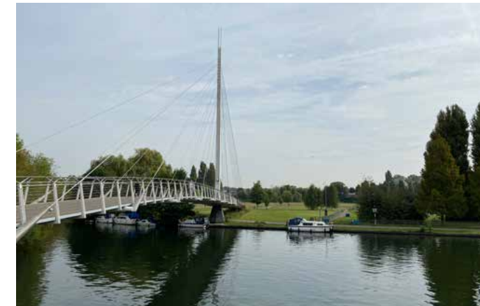
Photo 32: View from Thames Path towards Christchurch Bridge and Christchurch Meadows
