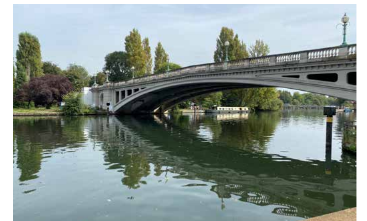
Photo 15: View north-east from Thames Path towards the River and Reading Bridge
