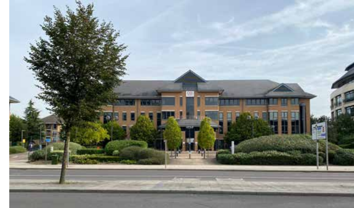
Photo 1: Site from Vastern Road
