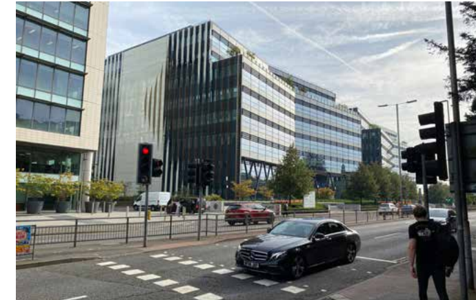
Photo 26: Two Forbury Place as seen from Forbury Road
