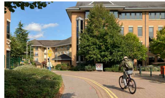
Photo 3: Western edge of the Site looking along Norman Place including the substation. Thames Court is seen beyond.
