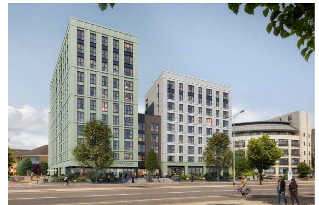
Frontage to Vastern Road
