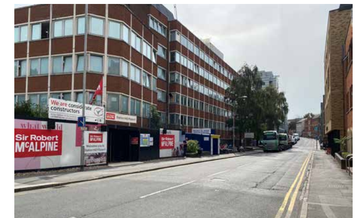
Photo 25: View south along Caversham Road
