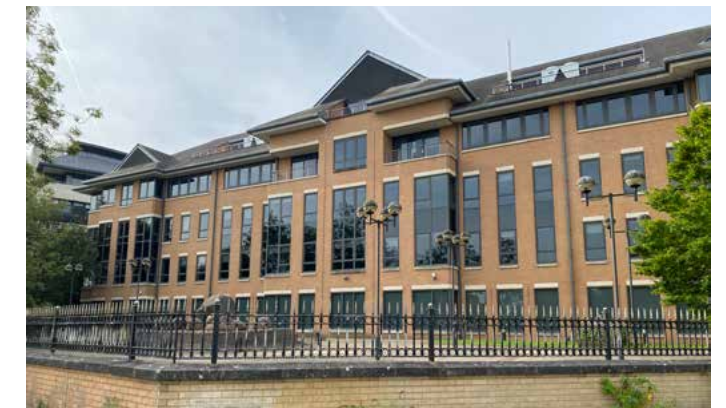
Photo 4: Site as viewed from the Thames Path
