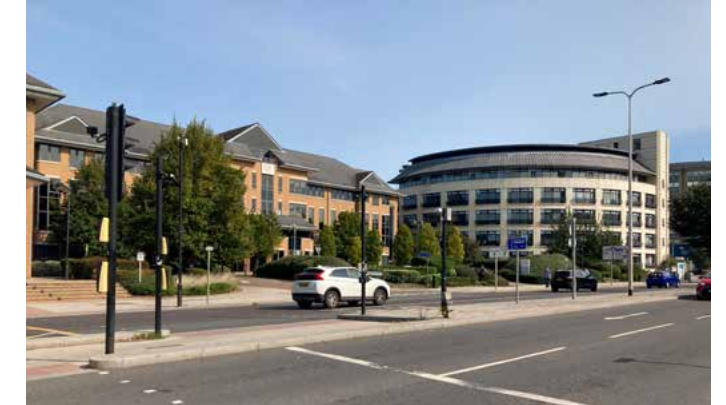
Photo 2: The site from from Vastern Road close to the junction with Trooper Potts Way
