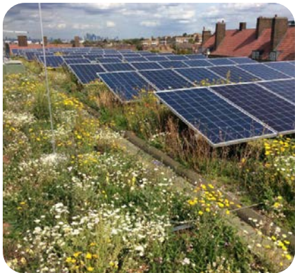
Biosolar green roof systems
