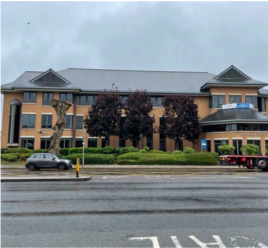
1. View from Vastern Road
