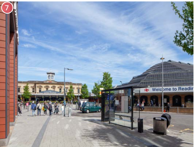
View from Station Road
