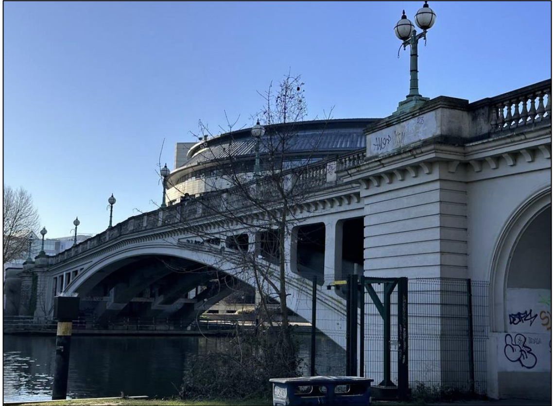
Figure 5.5 Reading Bridge from the north
