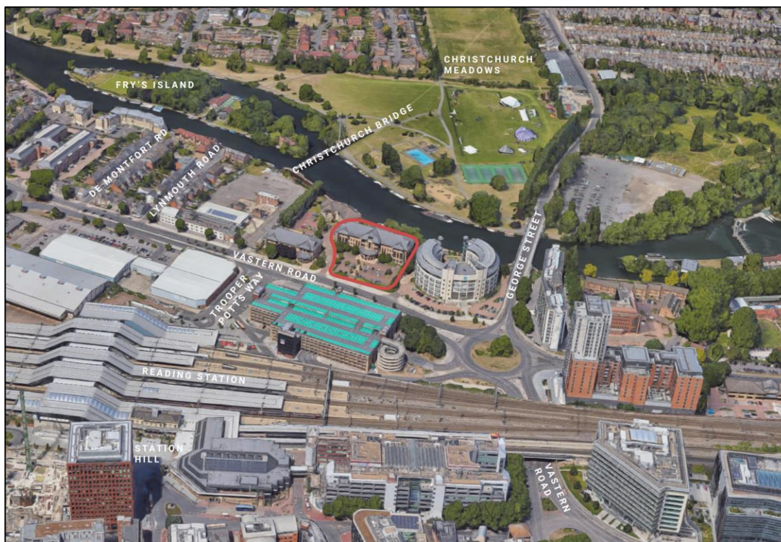
Figure 1.1 Aerial view of the site and surrounding context. Approximate site location outlined in red.
