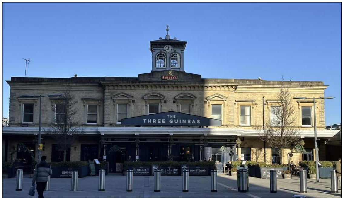
Figure 5.2 Main Building of Reading Station seen looking north towards the River Thames
