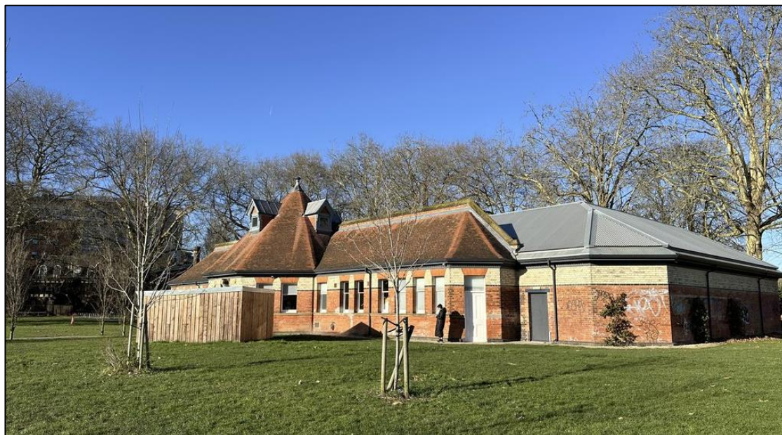
Figure 5.1 King's Meadow Swimming Pool Building, viewed from the south looking towards the site
