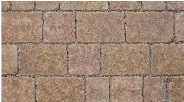
Rear parking bay from existing tarmac to paving
