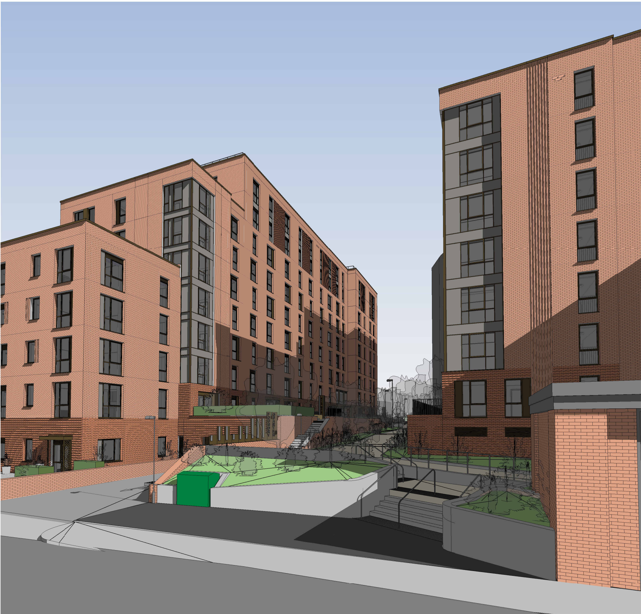
3 Central Pedestrian Way Looking South From Weldale Street
