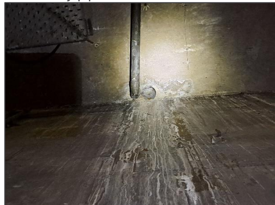
Photo 6. Showing a circular hole in the ceiling with water damage.
