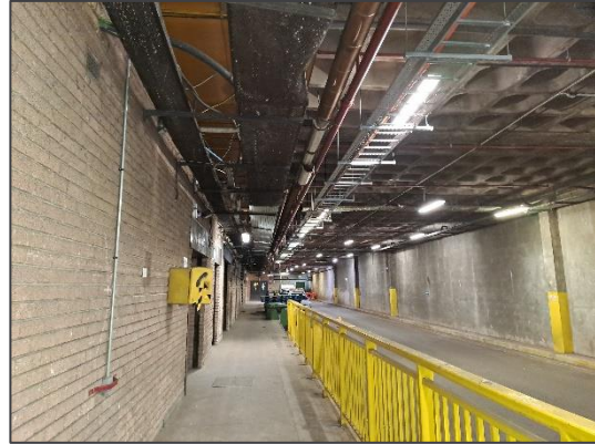
Photo 2. Showing the brightly lit central section of the service area
