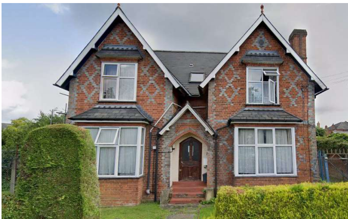
Figure 14. 83 Hamilton Road - Google Maps
