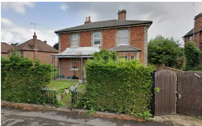
Figure 16. 81 Hamilton Road - Google Maps
