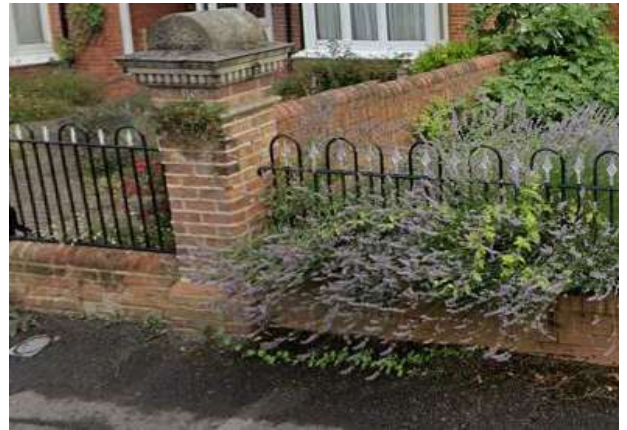
Figure 19. Brick and ironwork front boundaries
