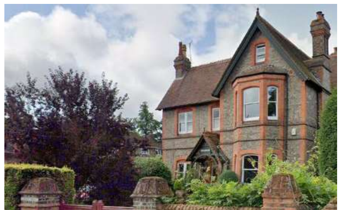
Figure 15. 120 Hamilton Road - Google Maps
