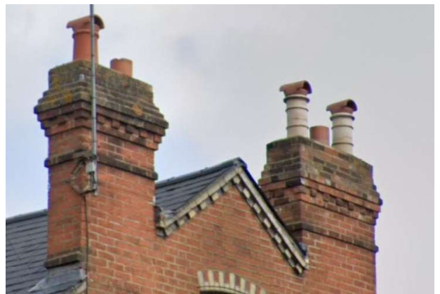
Figure 20. Large feature chimneys
