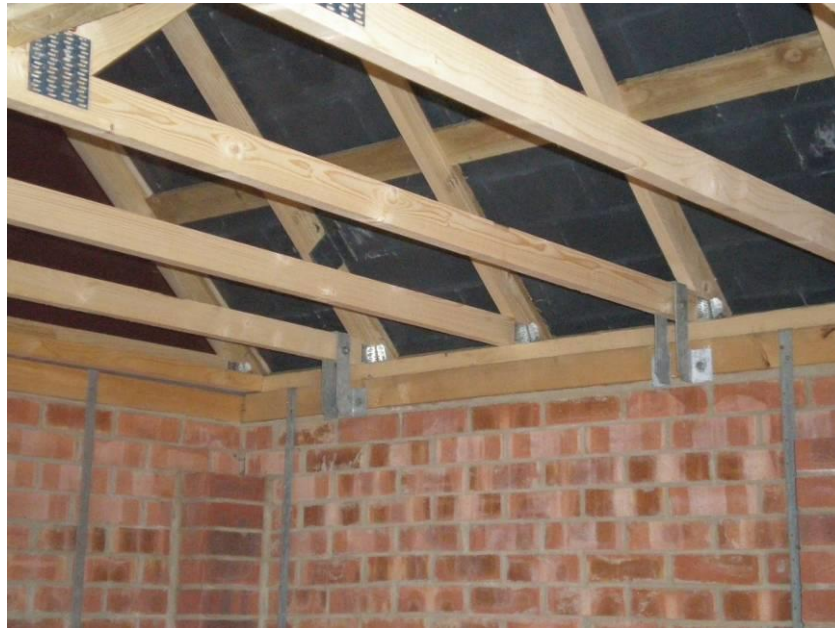
Photograph 3 - A separate wall plate is required. This shall be secured to the brickwork using restraining straps. The removable roof is secured to the wall plate using straps. The timber used for the trusses and wall plates shall be pressure treated with preservative.
