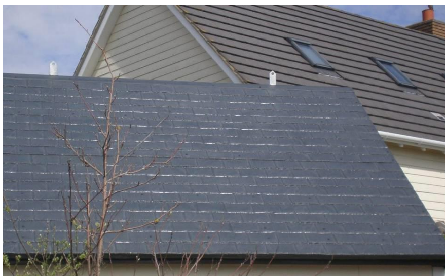
Photograph 2 - GRP roof showing lifting eyes.
