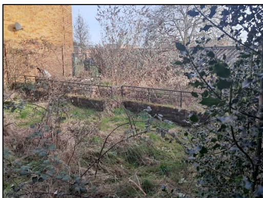
Figure 12: Mortared brick wall.
