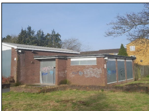
Figure 9: Eastern and north-eastern elevations of main on site building from the south-east.
