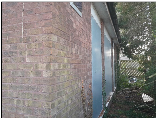
Figure 11: North-western corner elevation of main on site building from the north-west.
