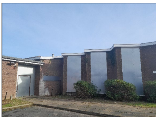
Figure 10: North-west elevation of main on site building from the south-west.
