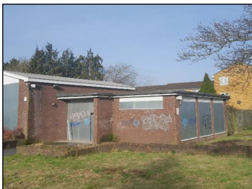
Figure 6: Eastern and north-eastern elevations of main on site building from the south-east.
