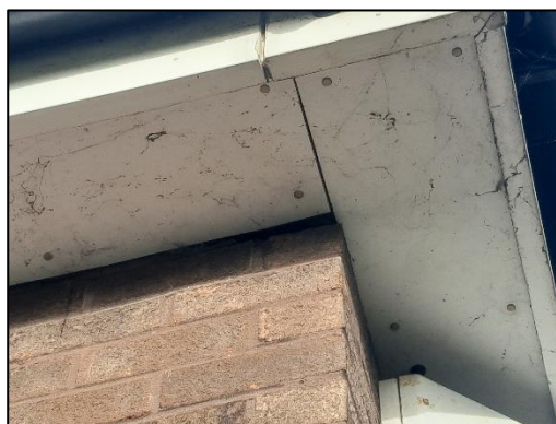
Figure 12: Gap behind soffit boxes on southern elevation of building.
