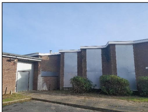
Figure 7: North-west elevation of main on site building from the south-west.
