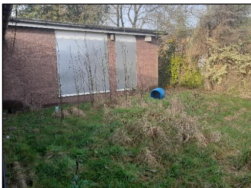
Figure 3: Area of tussocky modified grassland to the north of the building showing signs of a lack of management.
