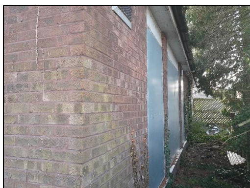
Figure 8: North-western corner elevation of main on site building from the north-west.
