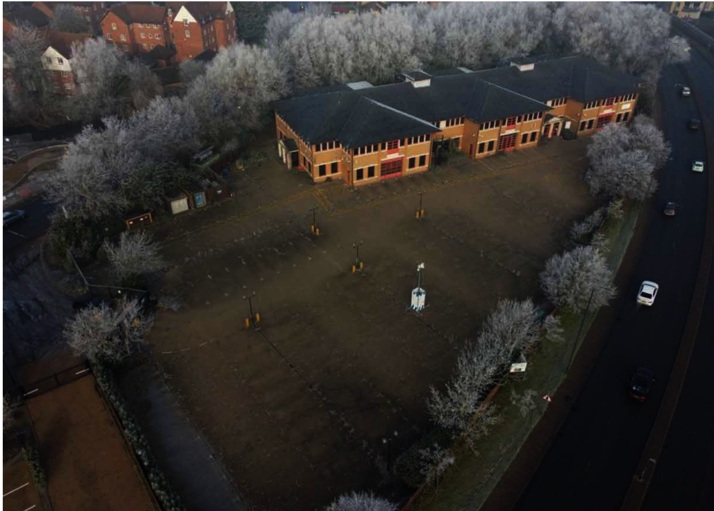
Fig. 5 Aerial View of Existing Site
