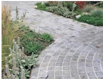
Driveway: Sandstone setts – light grey
