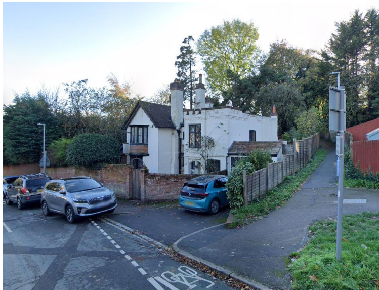
View from Surley Row onto the application site. Image taken from Google Maps on 09/09/2024.
