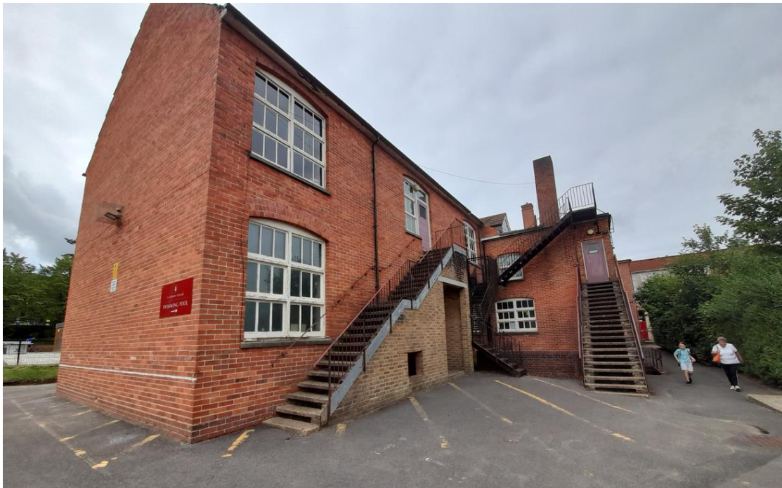
Fig. 13: View, looking south-west, of the east and north, rear elevations of B Block.
