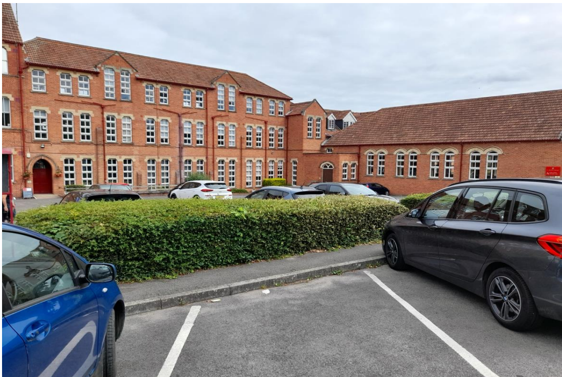
Fig. 14: View, looking north-east, of the middle range of school buildings and the adjoining former hall.
