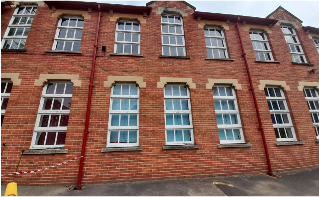
Fig. 12: View, looking south, of the south elevation of B Block, with details of fenestration.
