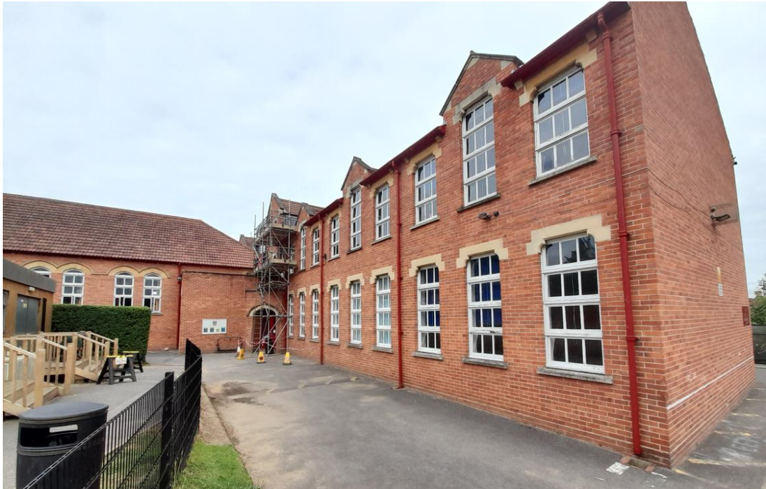
Fig. 19: View, looking north-west, of the south elevation and south-facing roof of B Block.
