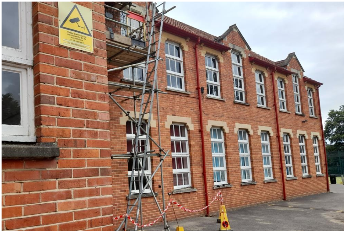
Fig. 11: View, looking north-east, of the south, front elevation of B Block.
