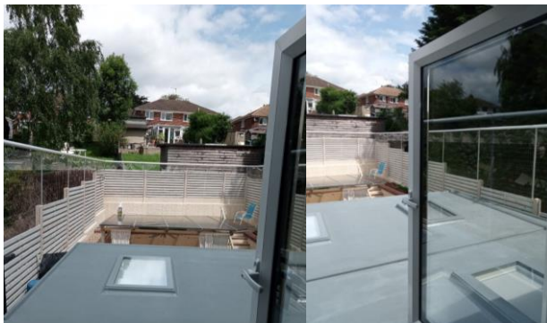
Looking towards the rear from the first floor
