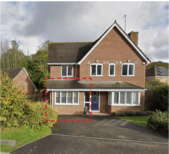
2 Treforgan Street elevation with converted garage indicated
