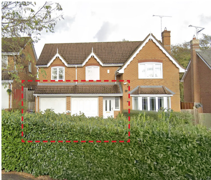
15 Hunters Chase Street elevation with indicated area to be converted
