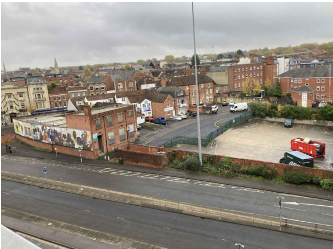
Plate 6: Overhead view looking south-east across the site from the multi-storey car park.
