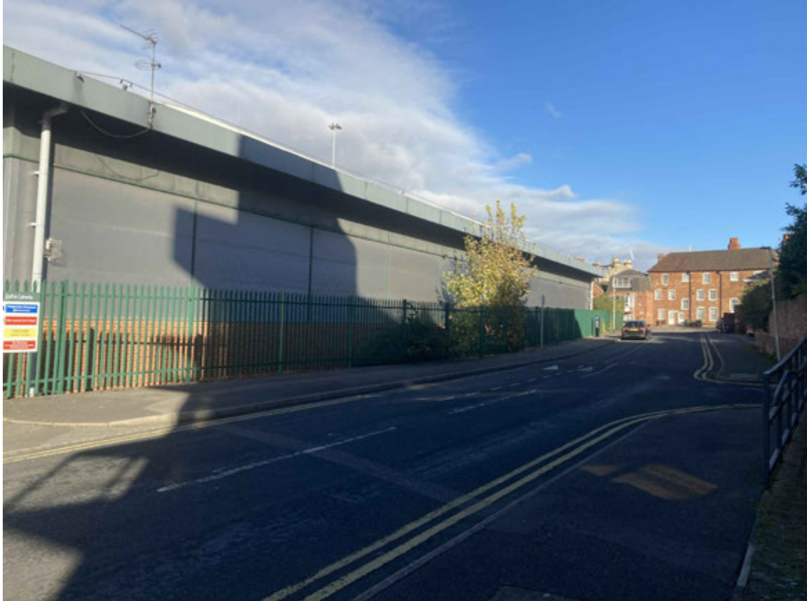
Plate 3: View from south of the site looking north-east
