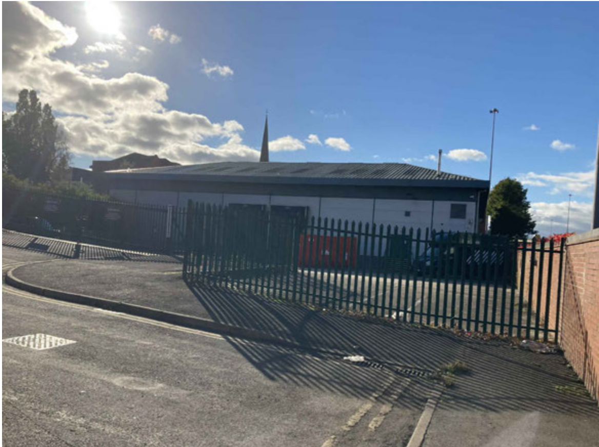
Plate 1: View from the north-east of the site looking south-west.
