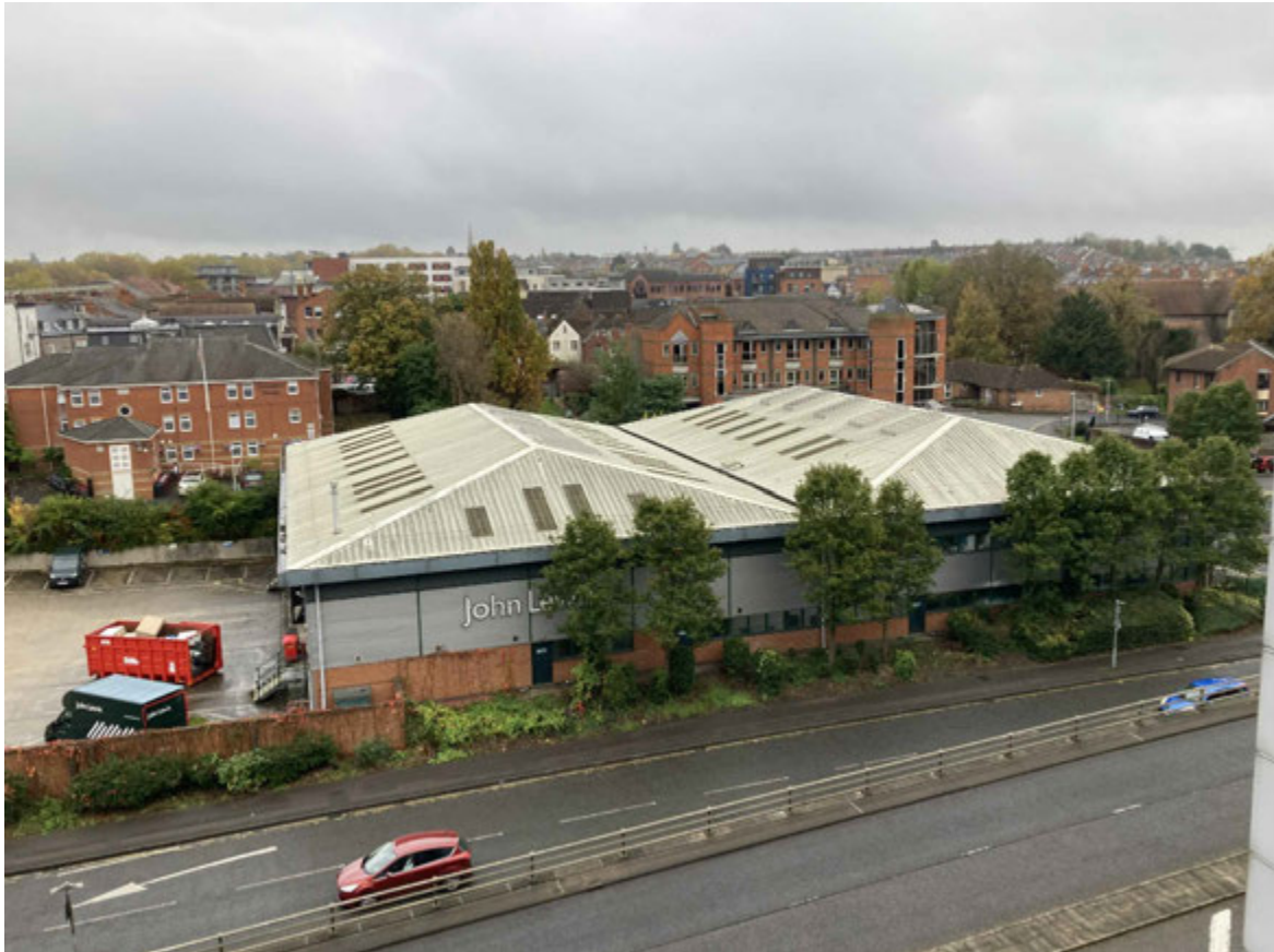
Plate 7: Overhead view looking south across the site from the multi-storey car park.
