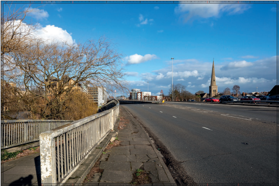
Figure 7.7 View 9: Bridge Street/A329 looking east. Source: Cityscape
