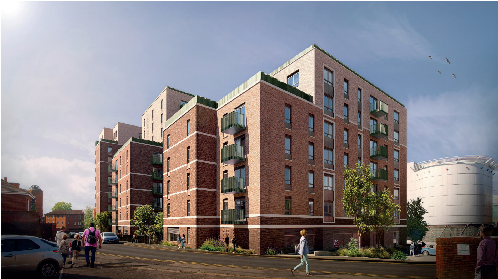
Figure 10.10 CGI showing the step down in height on the southern part of the Site. Source: DAS prepared by CJCT architects.
