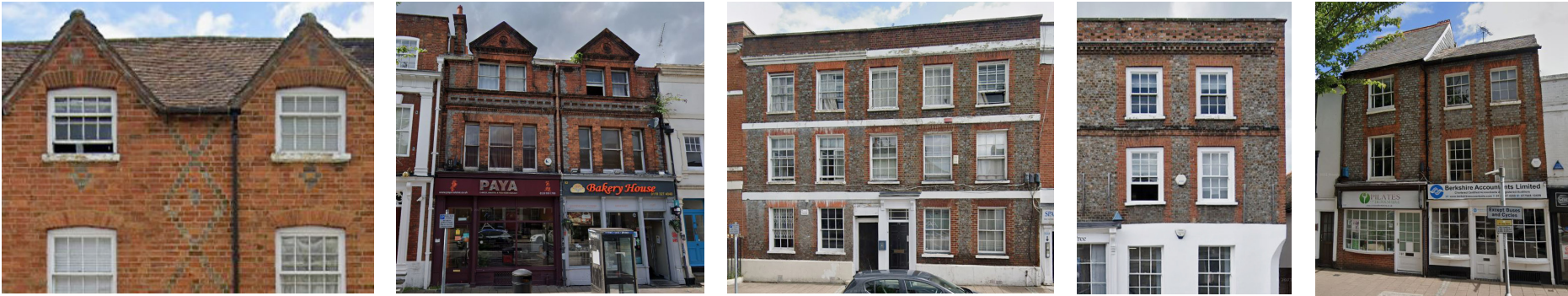
Grey and Red Brickwork Detailing
