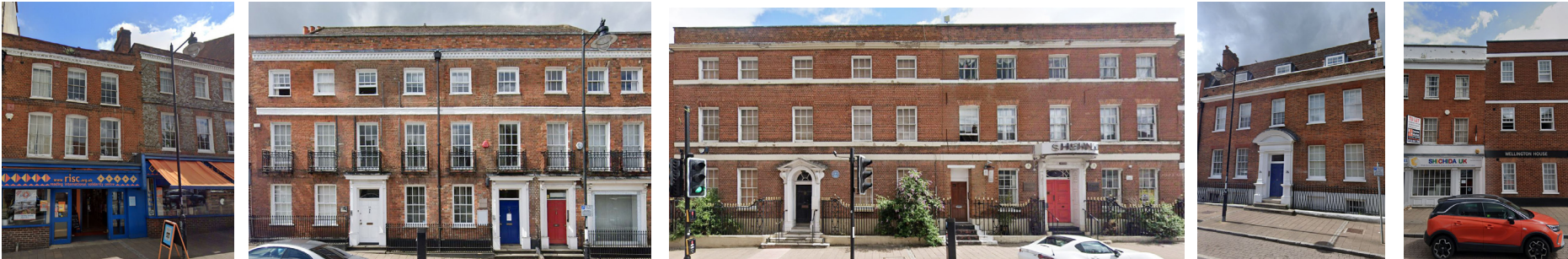
White Horizontal Banding and Cornice Detailing
