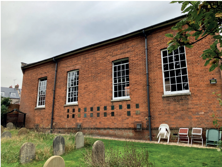
Figure 5.7 Rear elevation of the Quakers Meeting House
