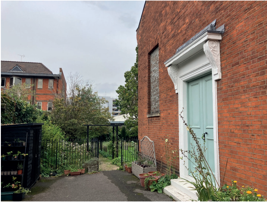
Figure 5.8 Main entrance to Quakers Meeting House and relationship with the burial ground to the north
