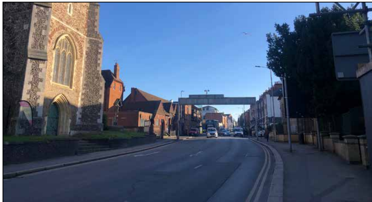
Figure 5.47 Showing LED luminaires mounted on approximately 8m high columns along Southampton Street looking south-east. Captured at approximate position of Survey Location A23
