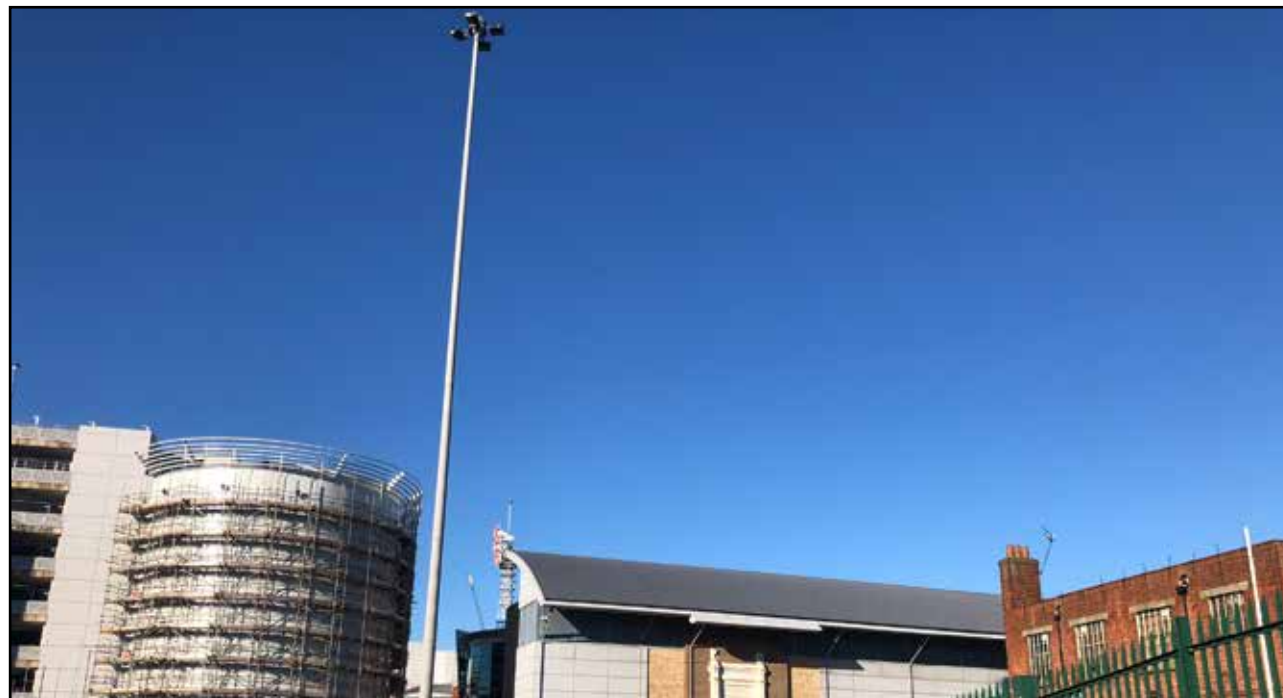
Figure 5.27 Showing luminaire mounted on 30 metre high column, looking north. Captured at approximate position of Survey Location A9.
