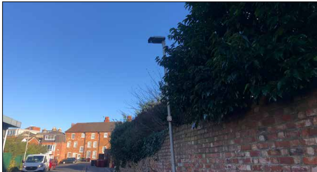
Figure 5.43 Showing LED luminaire mounted on approximately 6m high column along Crossland Road, looking east. Captured at approximate position of Survey Location A16.
