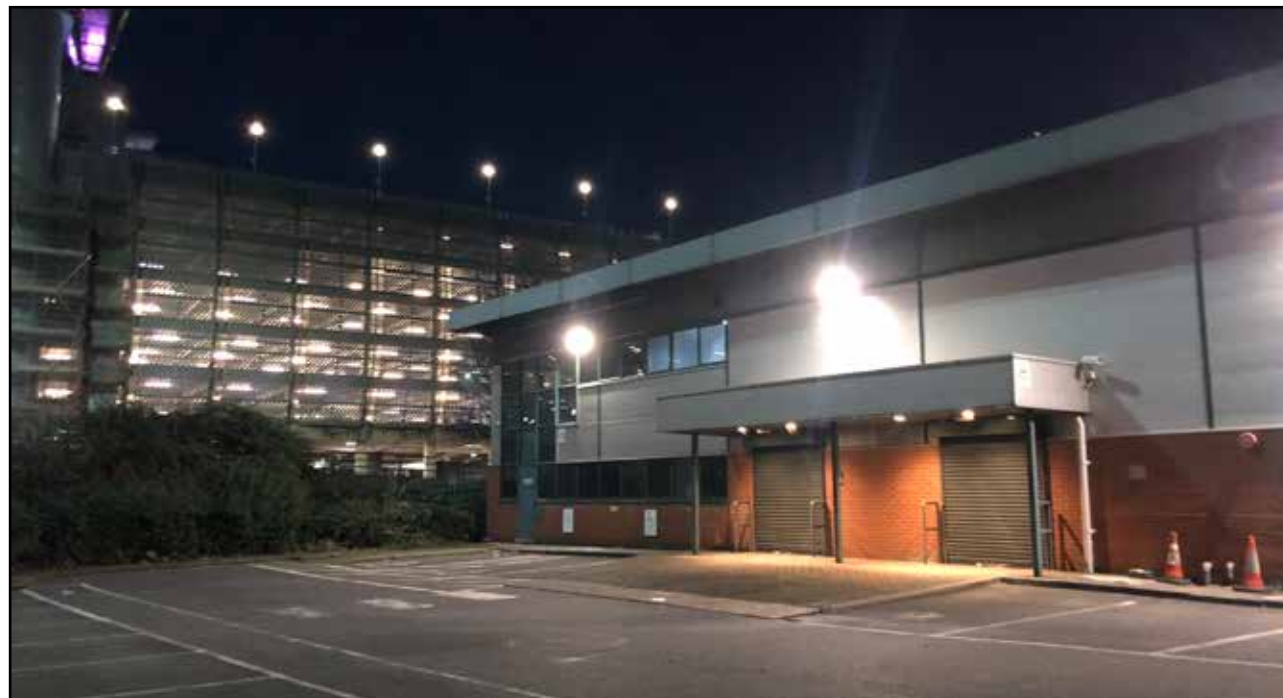
Figure 5.71 Showing building surface mounted floodlights on Site facade, looking north. MSCP in background. Captured at approximate position of Survey Location A19.
