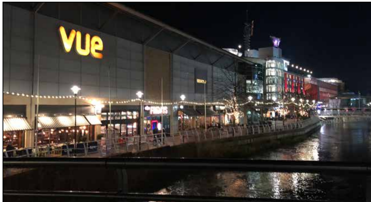
Figure 5.51 Showing LED luminaires mounted on approximately 6m high columns along Oracle Shopping Centre waterfront, looking south-west. Captured at approximate position of Survey Location A1.
