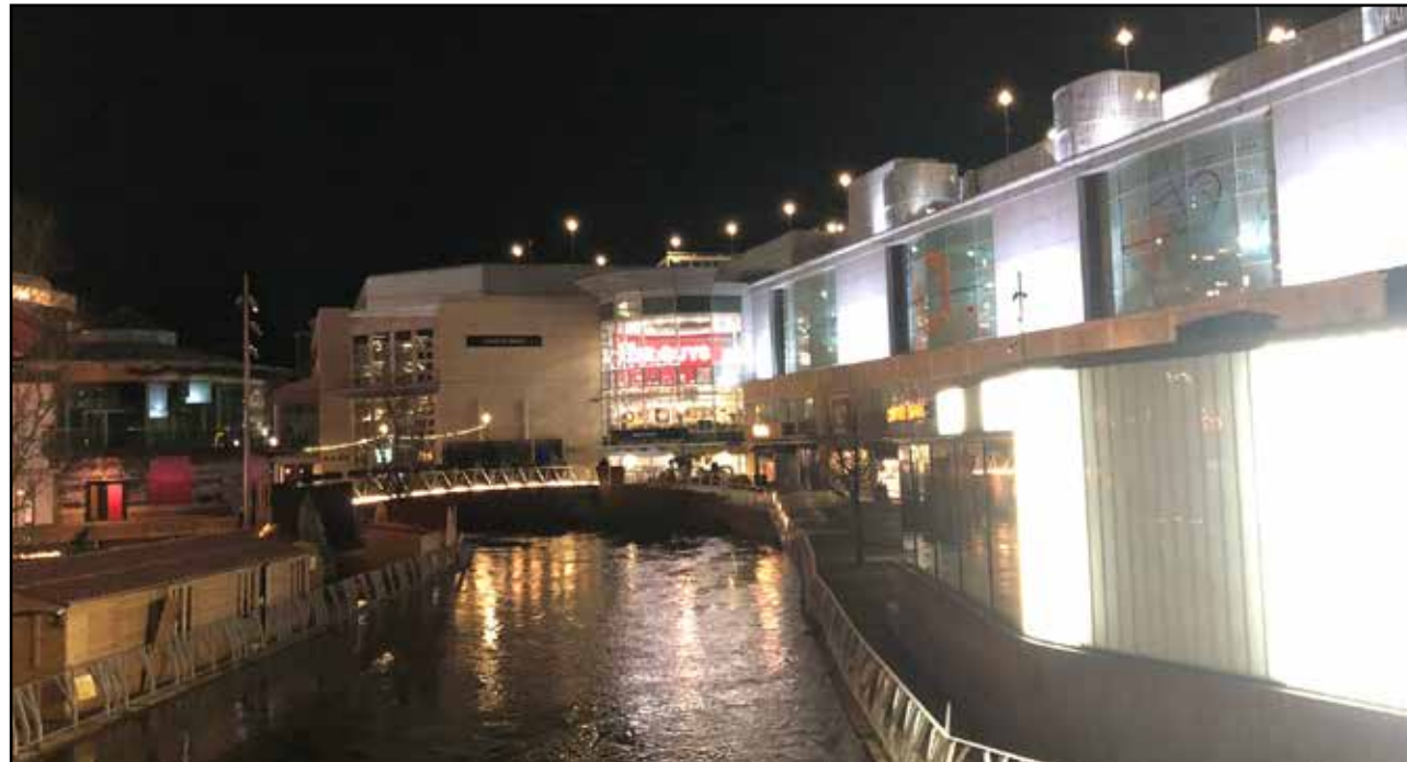
Figure 5.53 Showing illuminated branding/advertising installations of building frontages of Oracle shopping centre & River Kennet, looking south-west. Captured at approximate position of Survey Location A2.
