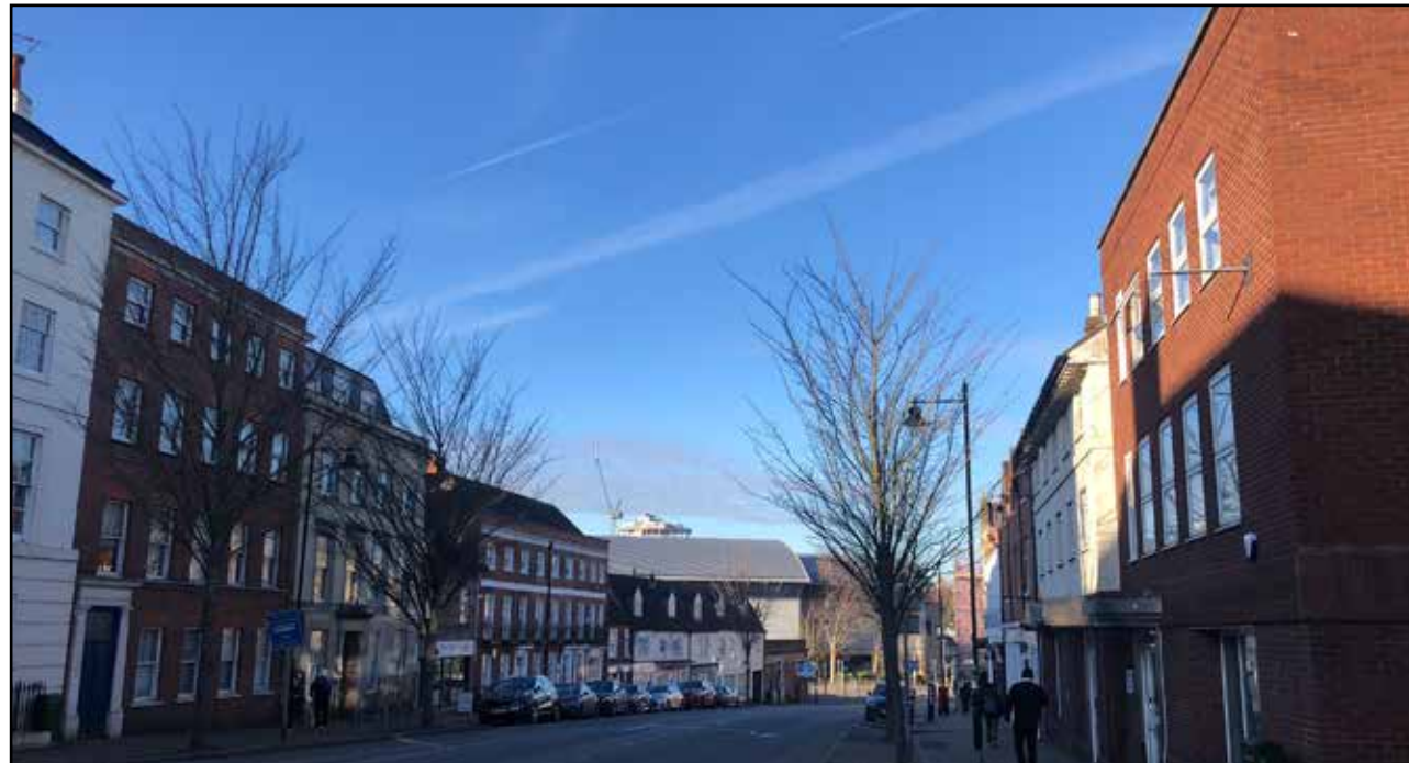
Figure 5.37 Showing luminaires mounted on approximately 6 metre high columns along London Street, looking north. Captured at approximate position of Survey Location A14.
