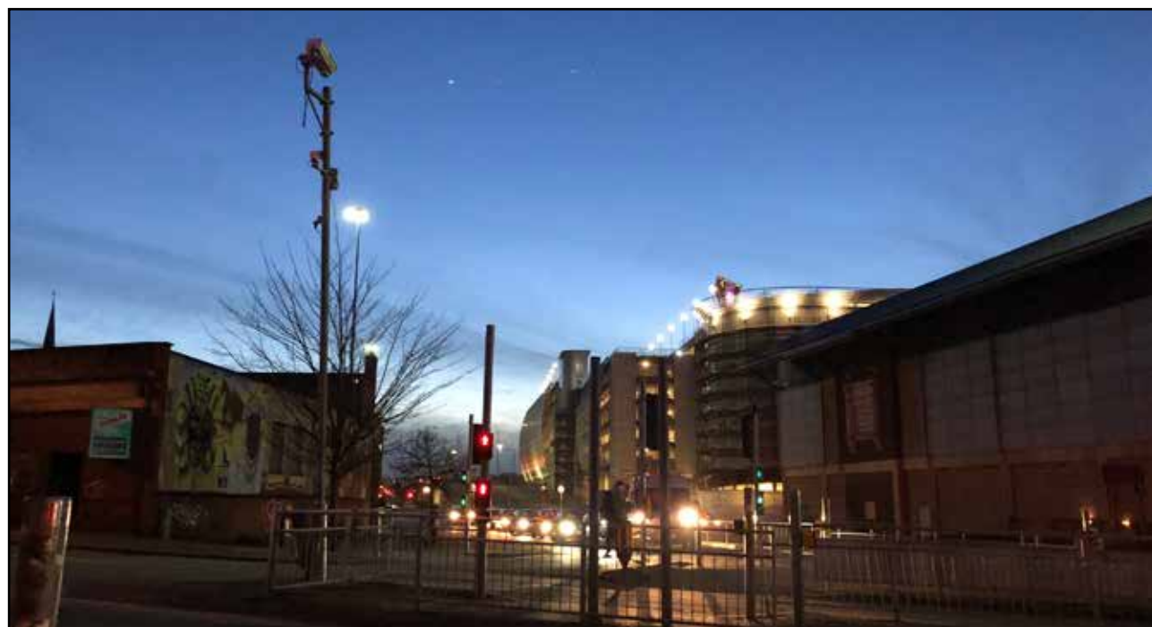
Figure 5.59 Showing luminaire mounted on 30 metre high column along A329/Mill Lane, looking south-west. Captured at approximate position of Survey Location A3.
