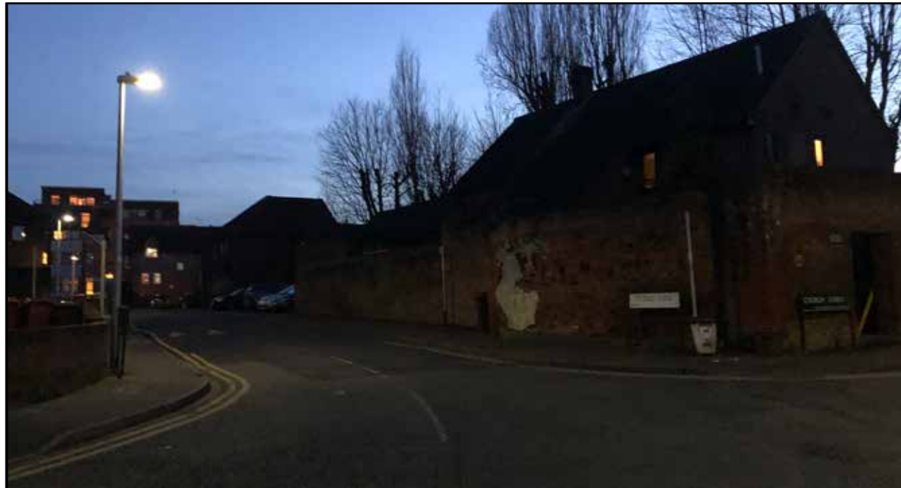
Figure 5.20 Showing LED luminaires mounted on approximately 6 metre high columns along Church Street, facing south-west. Townsend House on left of image. Captured at approximate position of Survey Location R4.
