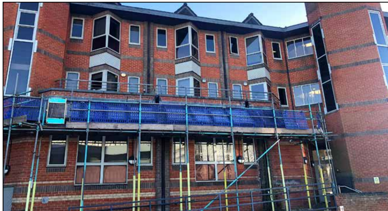
Figure 5.6 Showing bulkheads on Townsend House, looking south. Captured at approximate position of Survey Location R1.
