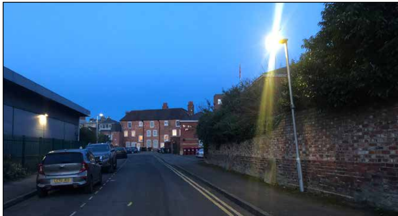
Figure 5.18 LED luminaires mounted on approximately 6 metre high columns along Crossland Road looking north-east. Reading Quakers Meeting House boundary on right. Captured at approximate position of Survey Location R1.
