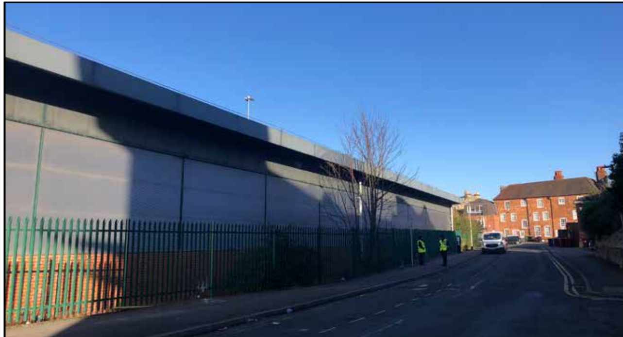
Figure 5.4 Showing LED luminaires mounted on approximately 6 metre high columns & building surface mounted floodlights, facing north-east. Captured at approximate position of Survey Location R1.
