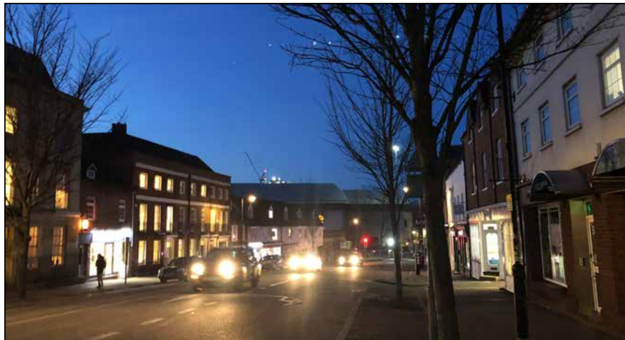
Figure 5.67 Showing luminaires mounted on approximately 6 metre high columns along London Street, looking south. Captured at approximate position of Survey Location A14.
