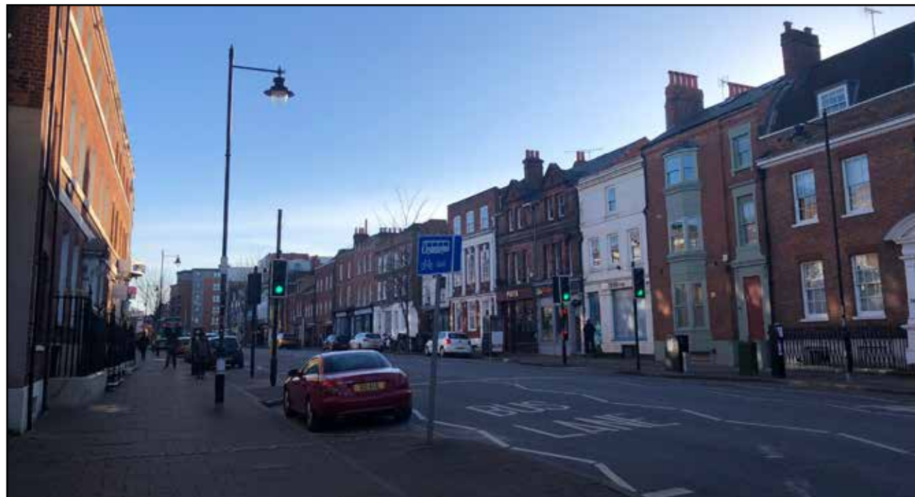
Figure 5.39 Showing luminaires mounted on approximately 6 metre high columns along London Street, looking south. Captured at approximate position of Survey Location A14.
