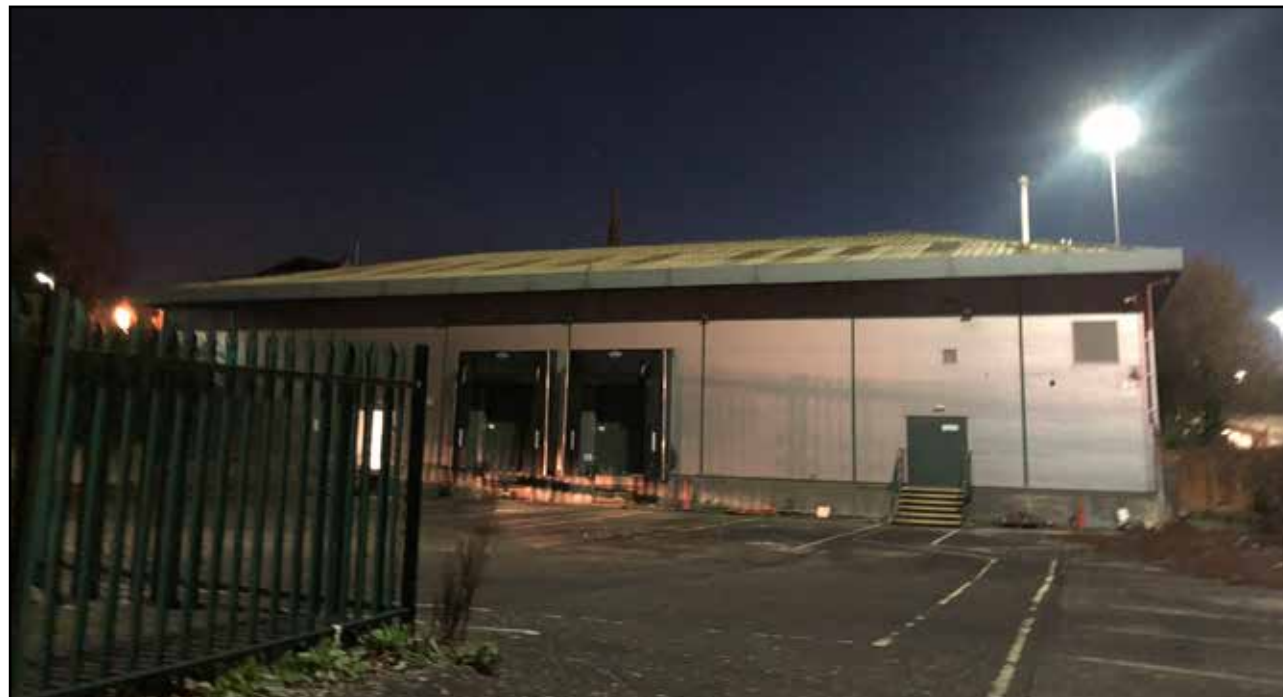
Figure 5.61 Showing loading bays with Site lighting switched off, looking south-west. Captured at approximate position of Survey Location A6.
