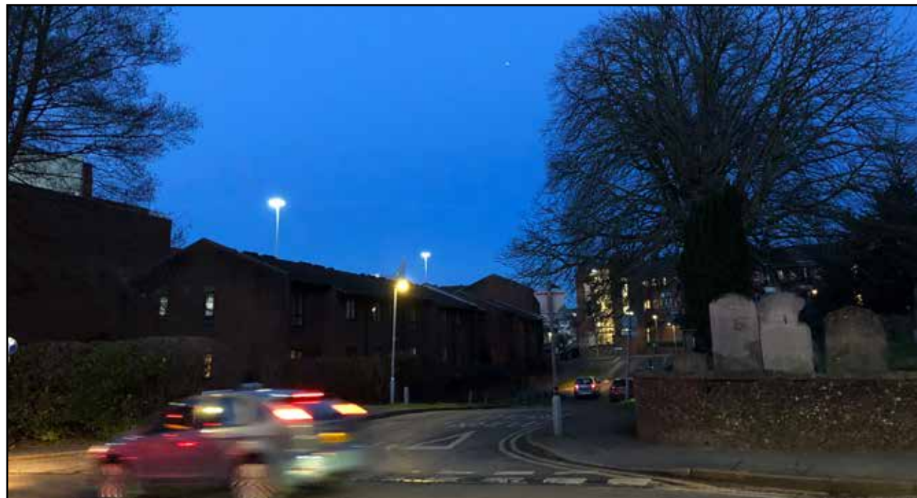
Figure 5.75 Showing luminaire mounted on approximately 6 metre high column along Deansgate Road, looking north-east. Site is middle/background. Captured at approximate position of Survey Location A23.
