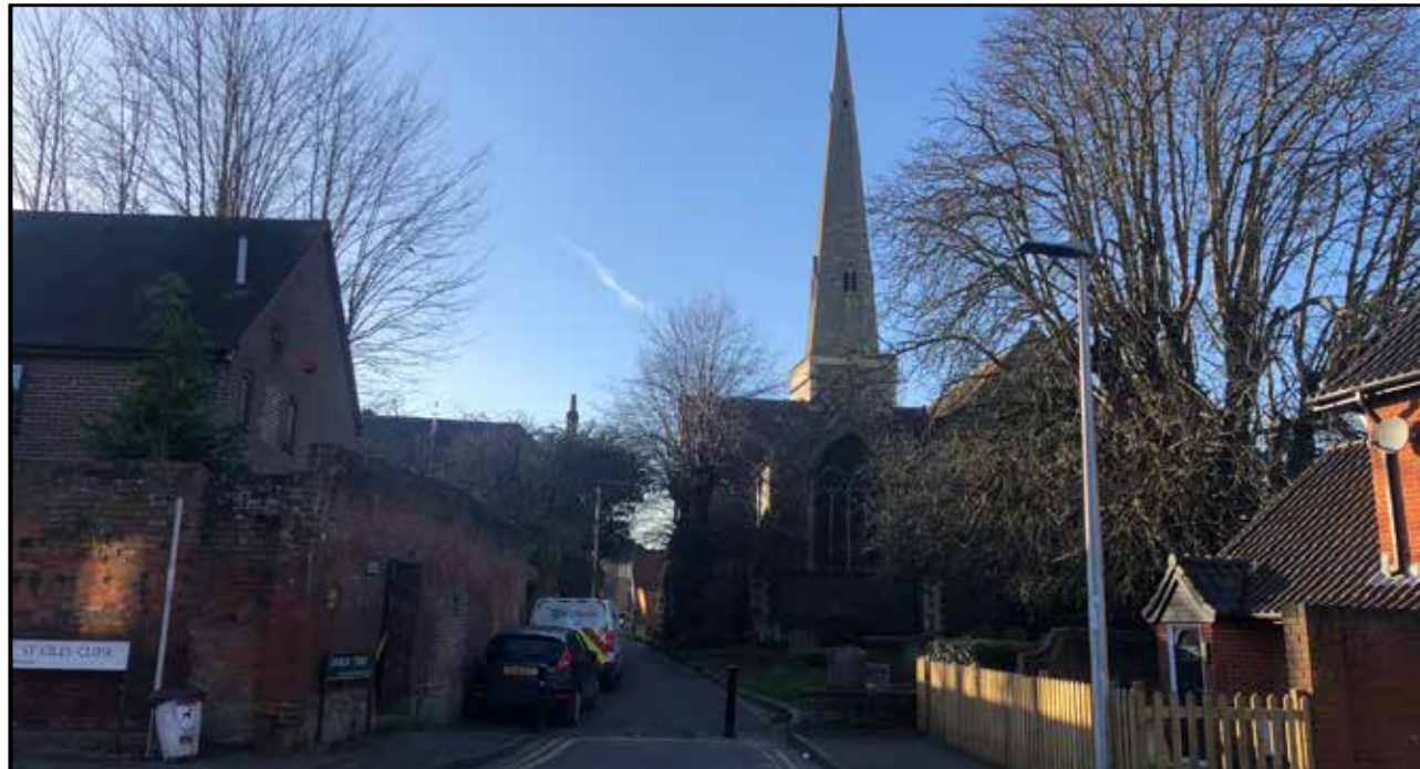
Figure 5.12 Showing LED luminaires mounted on approximately 6 metre high columns along St Giles Close, facing west. Captured at approximate position of Survey Location R4.
