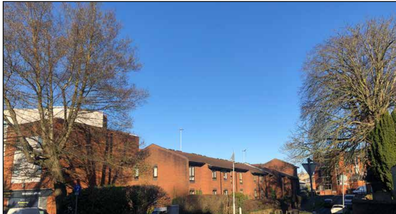
Figure 5.45 Showing LED luminaire mounted on approximately 6m high column along Deansgate Road looking north-east. Captured at approximate position of Survey Location A23.
