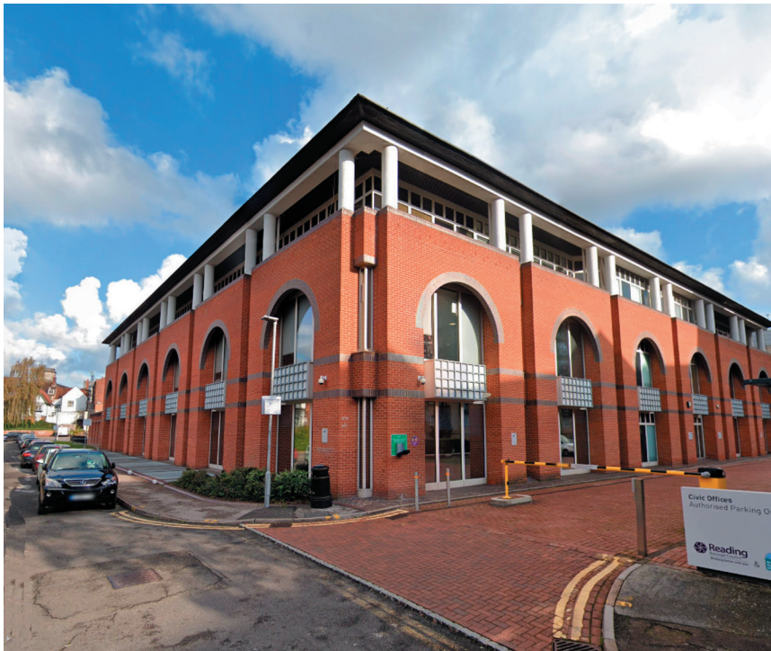
Reading Borough Council building
