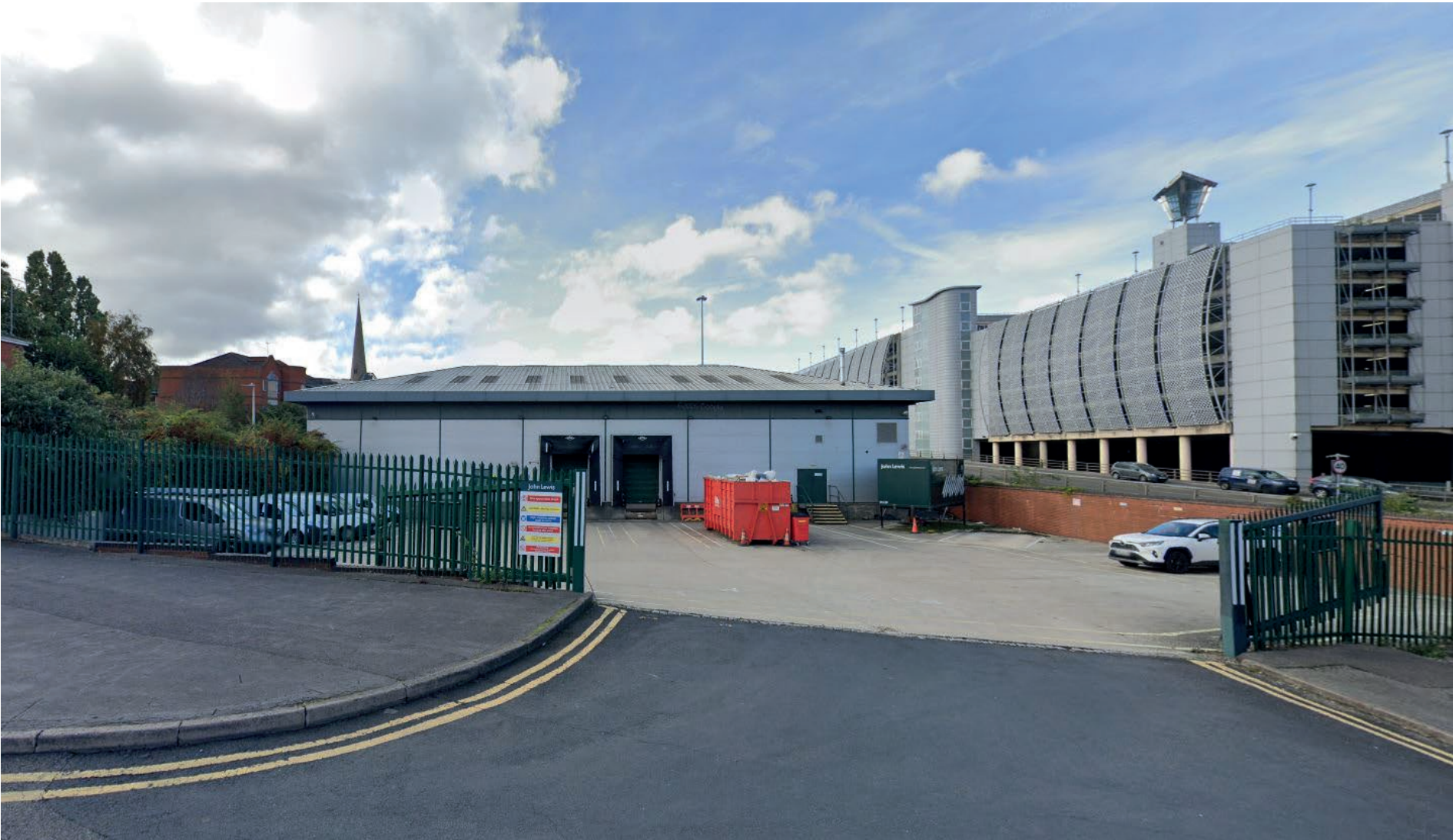
Figure 1.3 Current building on Site. Source: Google Street View October 2020.
