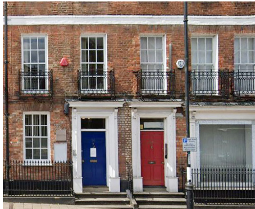
Horizontal banding, door surround
