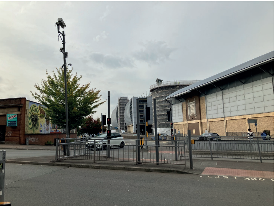
Figure 6.2 The Oracle Shopping Centre and associated multi-storey car park on the northern side of the IDR.
