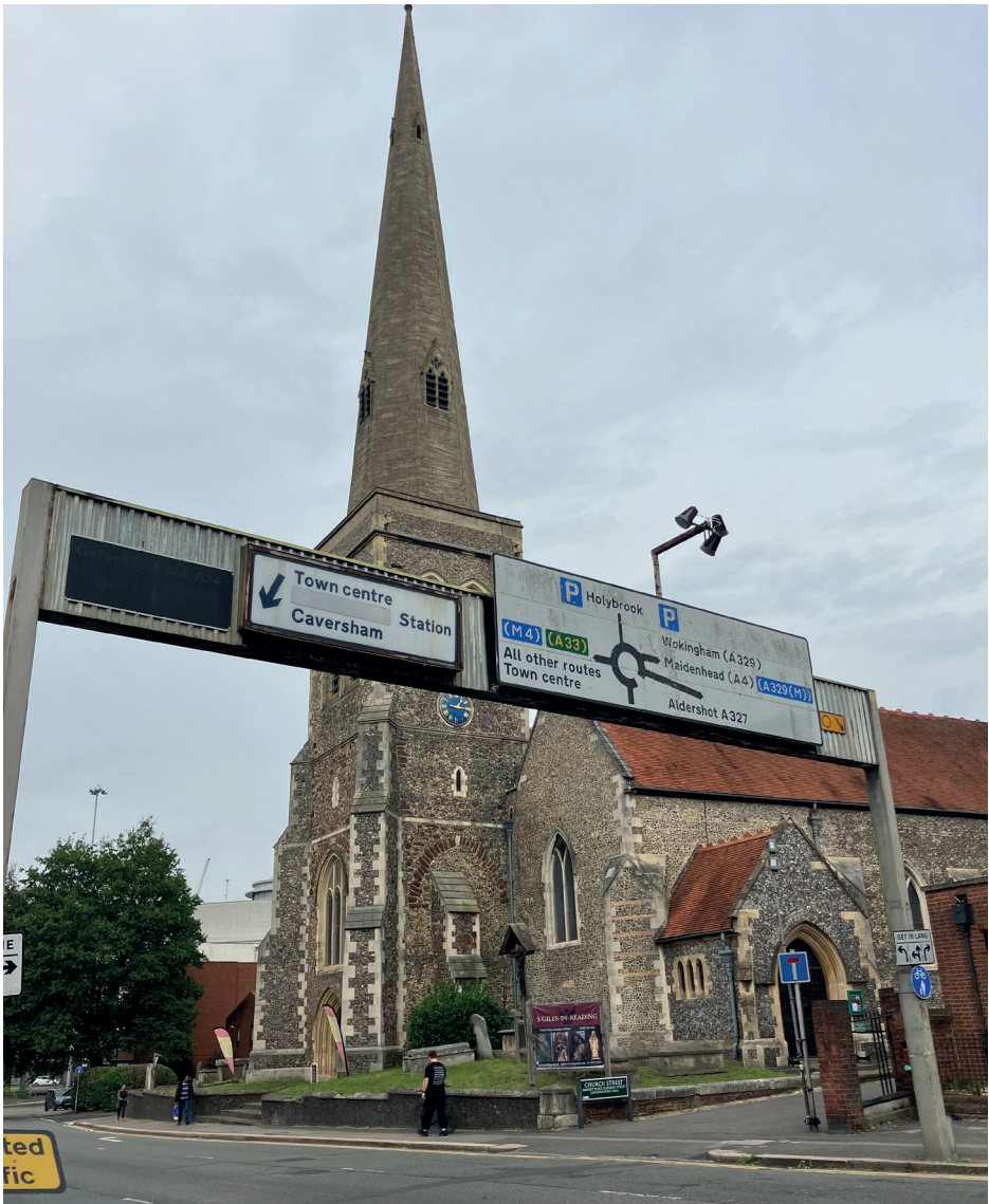
Figure 5.12 Road signage in front of the Church of St Giles
