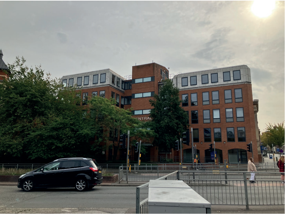
Figure 6.3 Commercial development on the southern side of the IDR.
