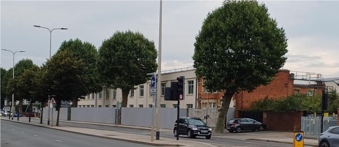
Site photograph 28/08/2024, showing the hoarding already in place (but no advertisement is displayed), with two inset areas to accommodate existing street trees.
